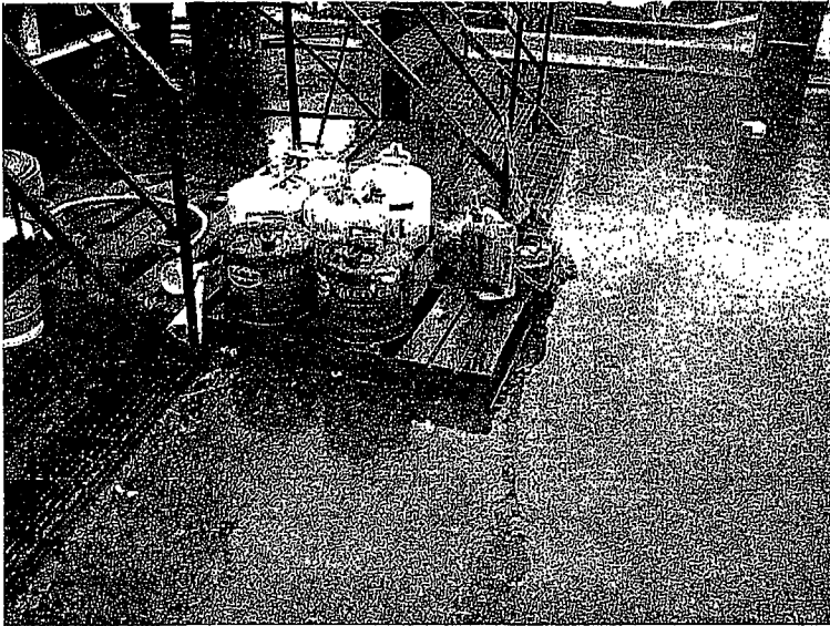
167. Gasoline storage has inadequate cover or containment to minimize storm water exposure.
