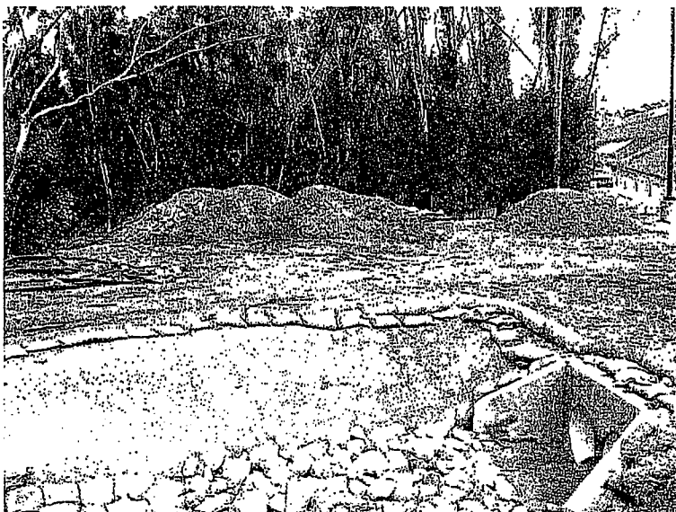
210. Soil stockpiles near Carroll Canyon Creek do not have cover or containment.
