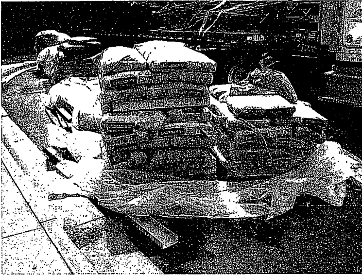
182. Bags of lime left out in the rain without cover.
