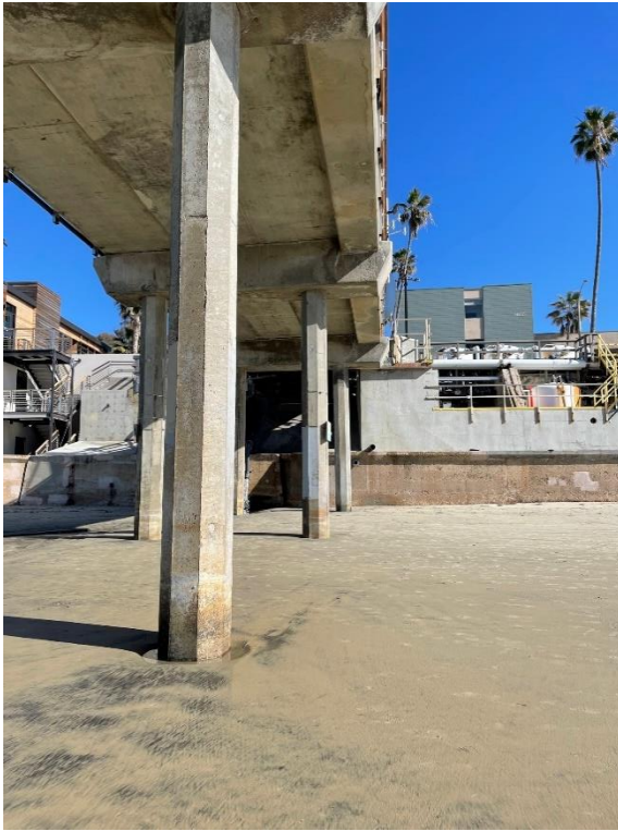
Photo 7: Photo provided by Kimberly O' Connell of University of California San Diego on February 8, 2023, showing bottom of the pier. Note that there is no sand displacement or loss below the pier.
