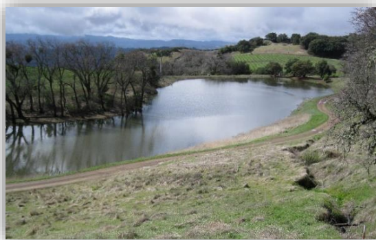
Photo by: State Water Board staff.
