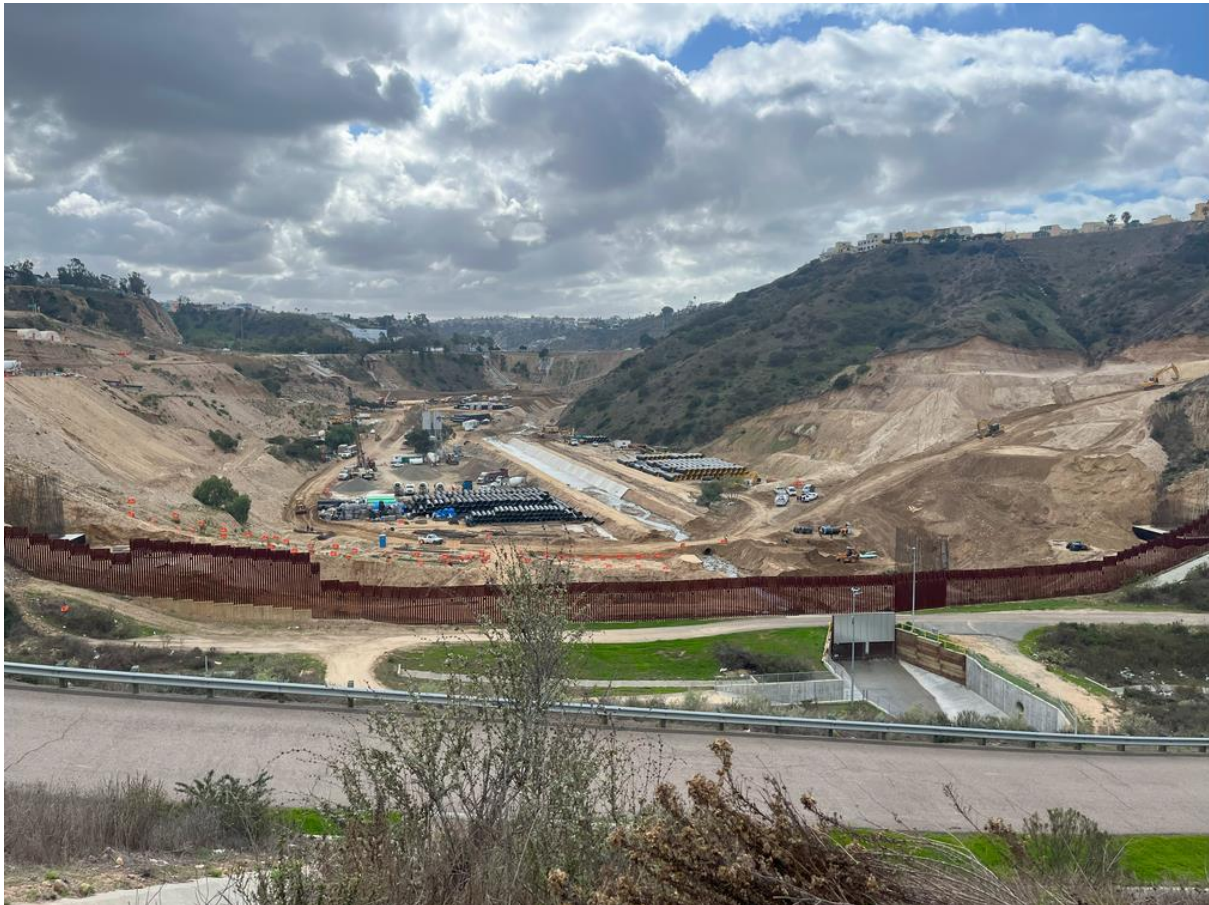
Figure 11: Mexican construction project in Matadero Canyon. (MC 01/10/2024)
