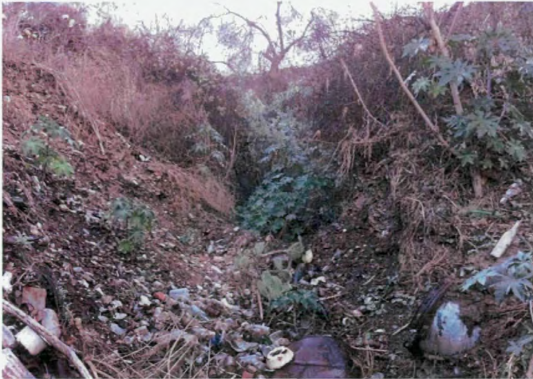
Photograph 3: Photo depicts upstream view of the drainage feature from the approximate midpoint of the proposed project.
