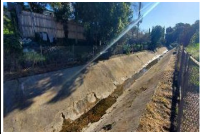
Cowles Mountain 2 Post-Maintenance- Photo 2
