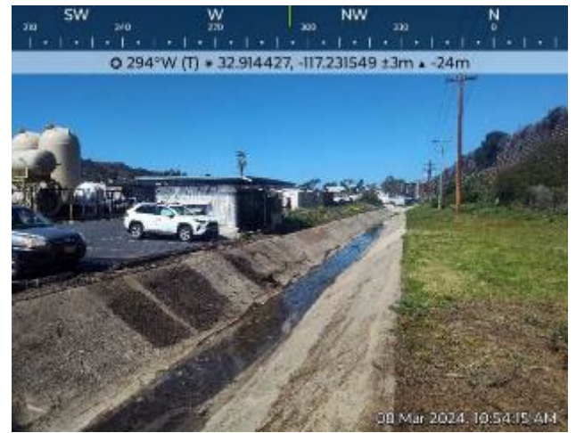
Tripp 1 Post-Maintenance- Photo 2
