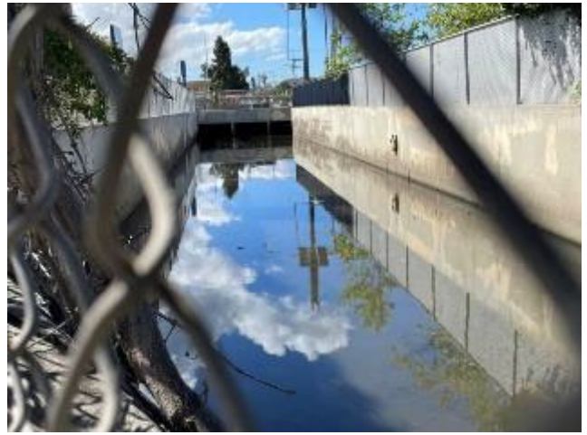
Cedar 2 Post-Maintenance- Photo 2
