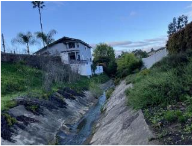
Cowles Mountain 1 Pre-Maintenance- Photo 1
