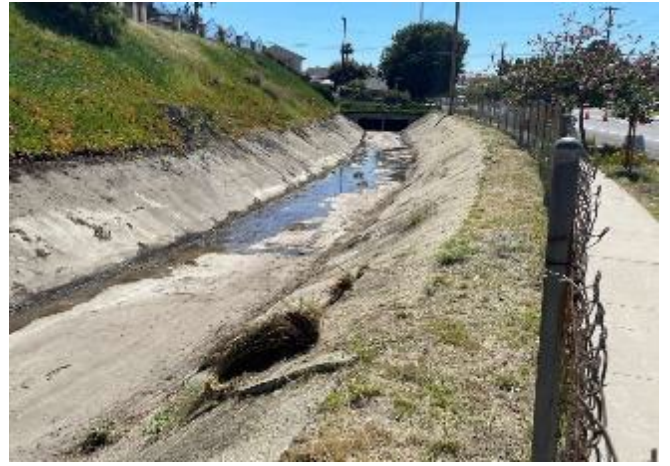
Parkside 1 Post-Maintenance- Photo 2
