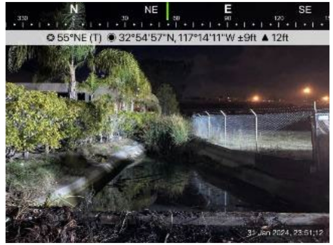
Industrial 2 Post-Maintenance- Photo 2
