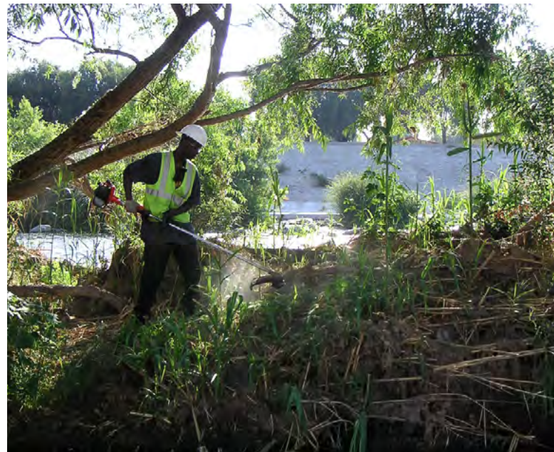
Figure 153. A worker removes invasive plant material from the channel near the Glendale Narrows, a maintenance practice that helps to increase the flood capacity of the LA River. Source: US Army Corps of Engineers, LA River Arundo Removal, 2004.
