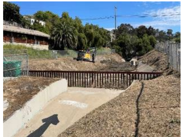
Washington 1 Post-Maintenance- Photo 2
