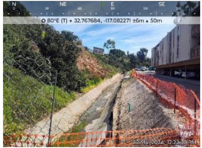
Baja 1 Post-Maintenance- Photo 2
