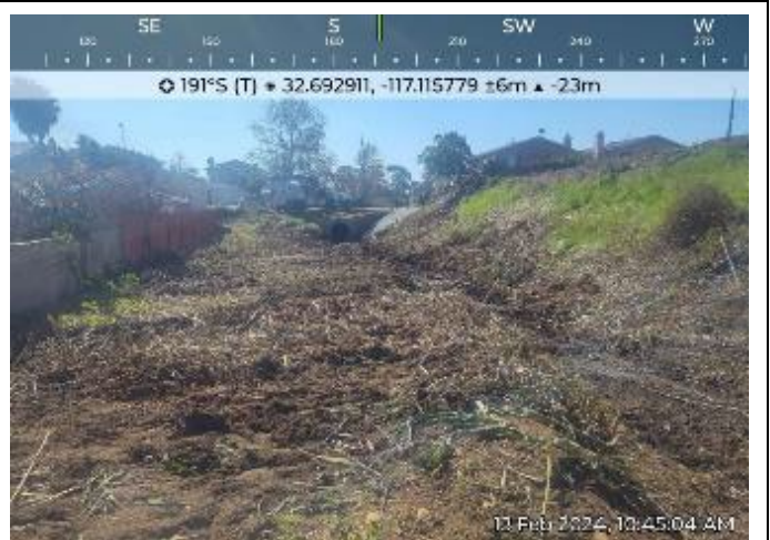
Acacia Grove 2 Post-Maintenance- Photo 2
