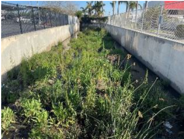
Cedar 2 Pre-Maintenance- Photo 1
