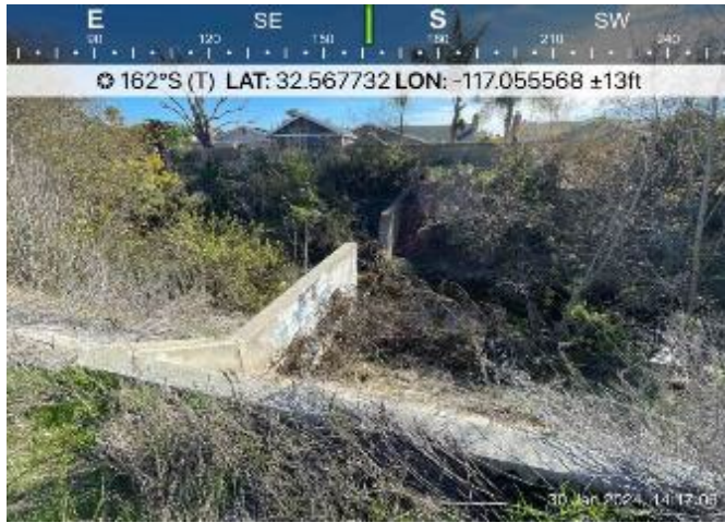
Smythe 1 Pre-Maintenance- Photo 1
