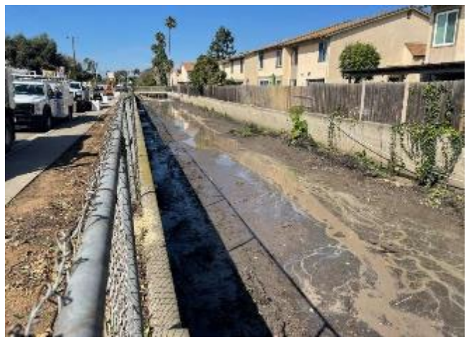
Grove 1 Post-Maintenance- Photo 2
