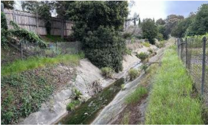
Cowles Mountain 2 Pre-Maintenance- Photo 1
