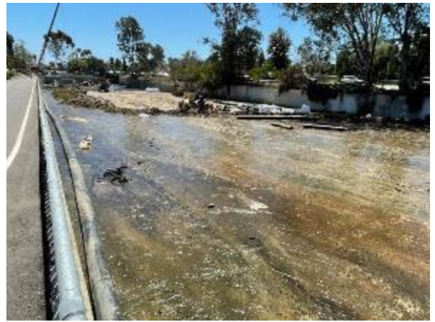
Damon 1 Post-Maintenance- Photo 2
