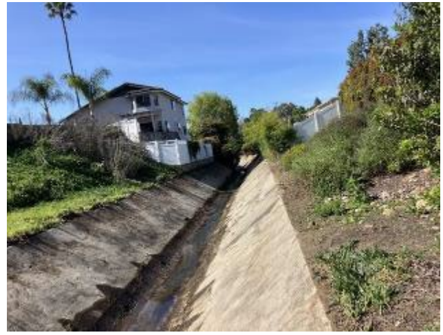
Cowles Mountain 1 Post-Maintenance- Photo 2
