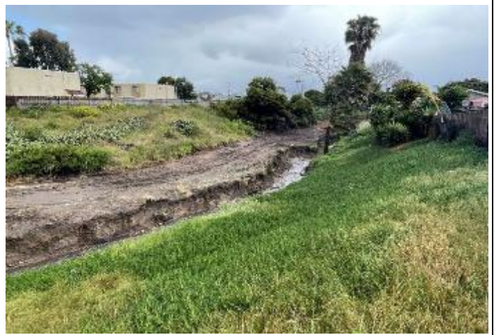
Castana 1 Post-Maintenance- Photo 2
