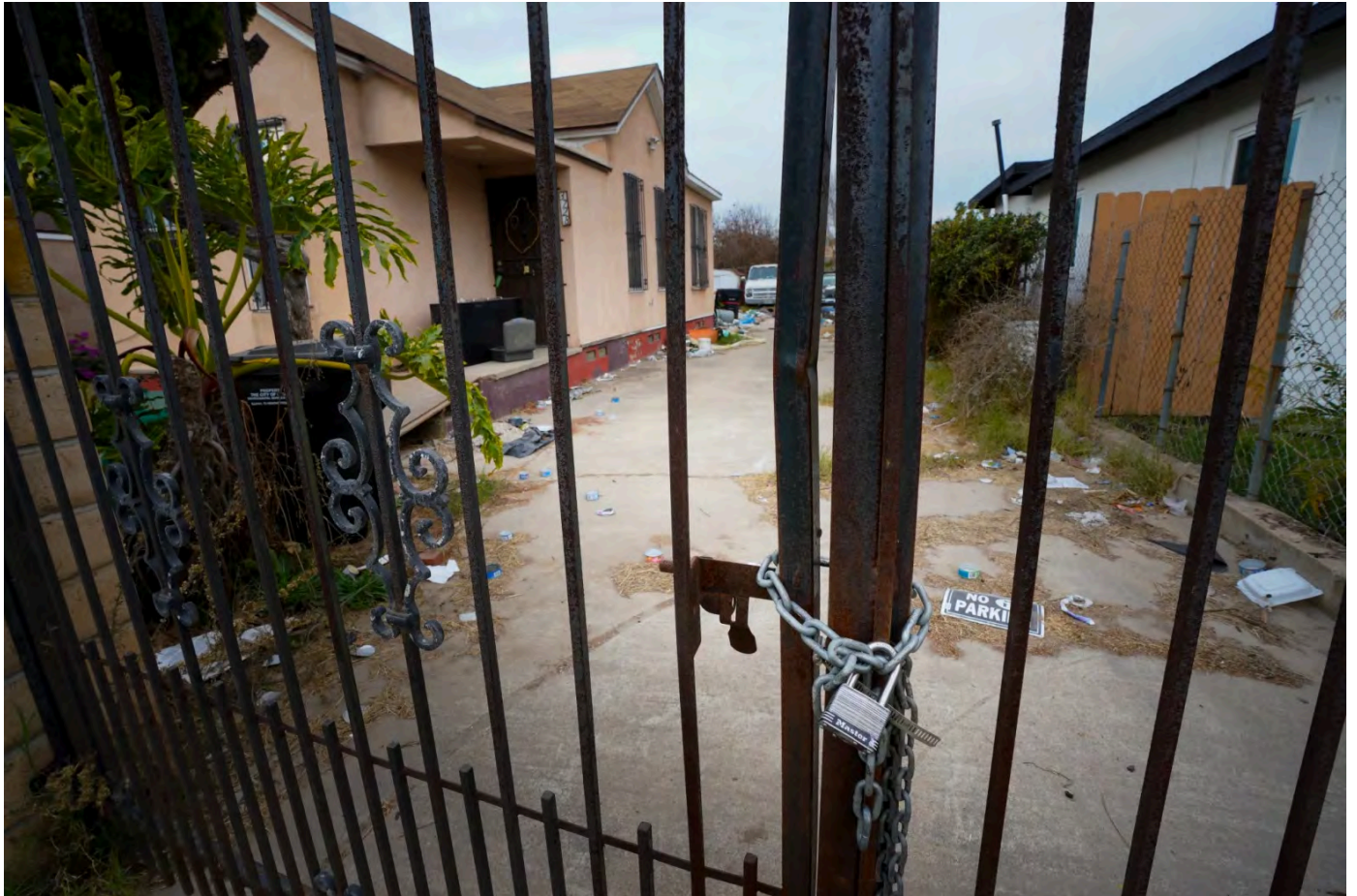
Almost a year later, this home on Beta Street shows very little sign of construction repairs from flood damage in the Southcrest community. (Nelvin C. Cepeda / The San Diego Union-Tribune)
