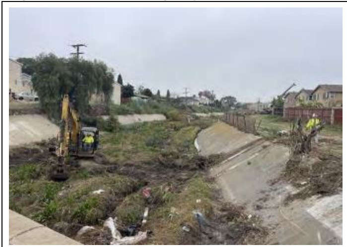
Alpha 1 Pre-Maintenance- Photo 1
