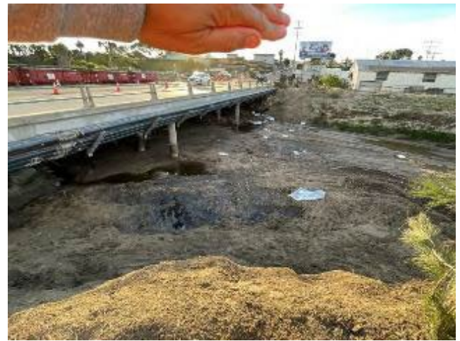
National 1 Post-Maintenance- Photo 2
