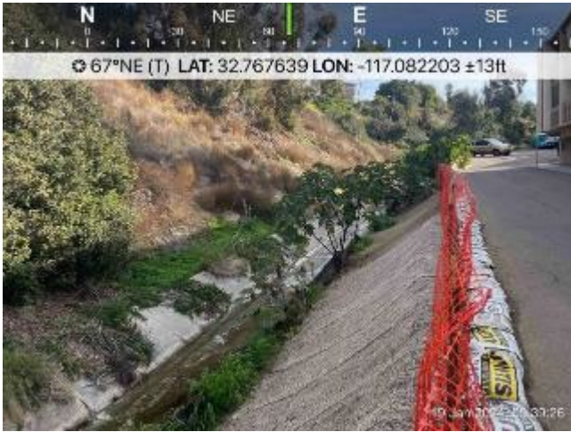
Baja 1 Pre-Maintenance- Photo 1
