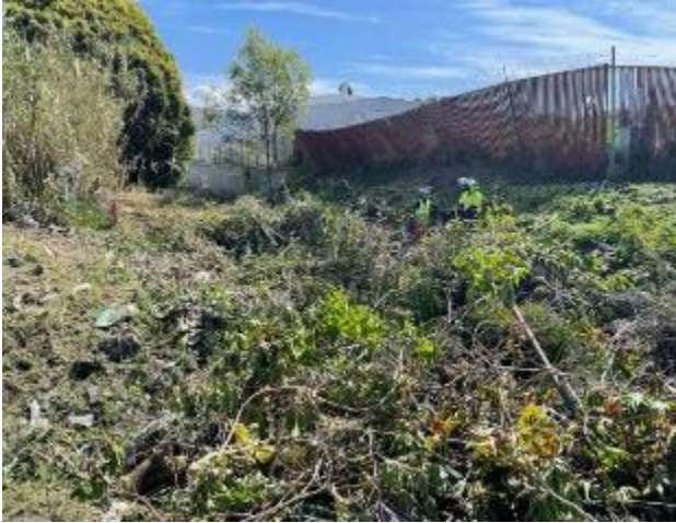
Cedar 1 Pre-Maintenance- Photo 1
