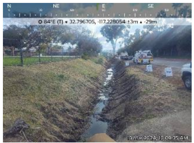
PB Olney 1 Post-Maintenance- Photo 2
