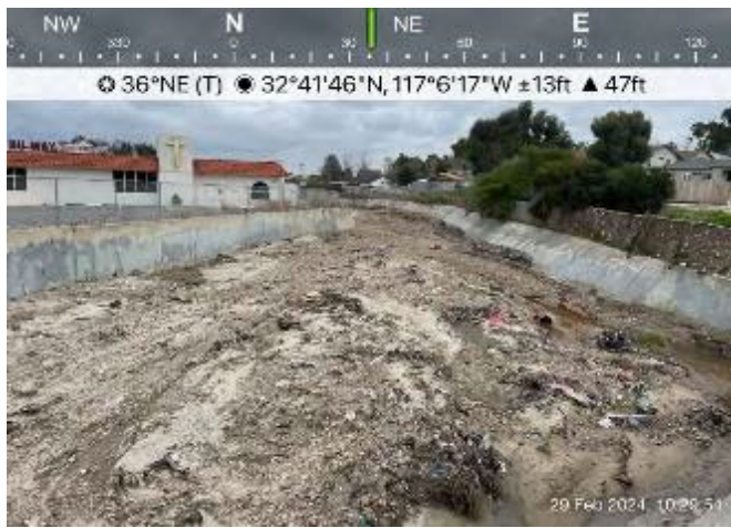
Ocean View 1 Pre-Maintenance- Photo 1
