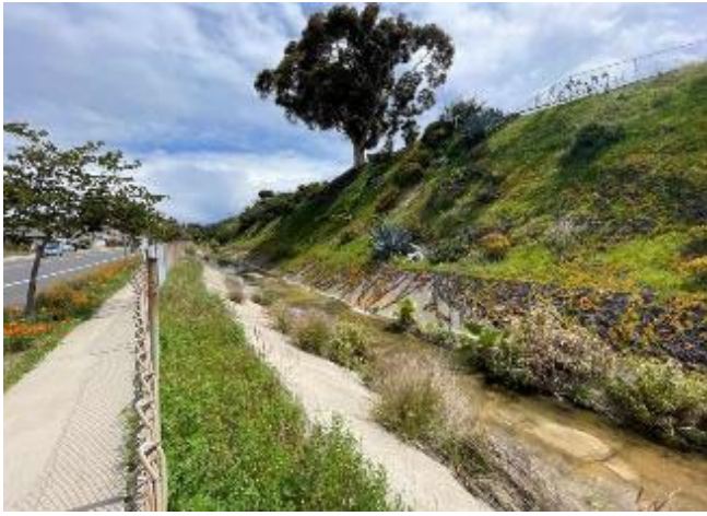
Parkside 1 Pre-Maintenance- Photo 1
