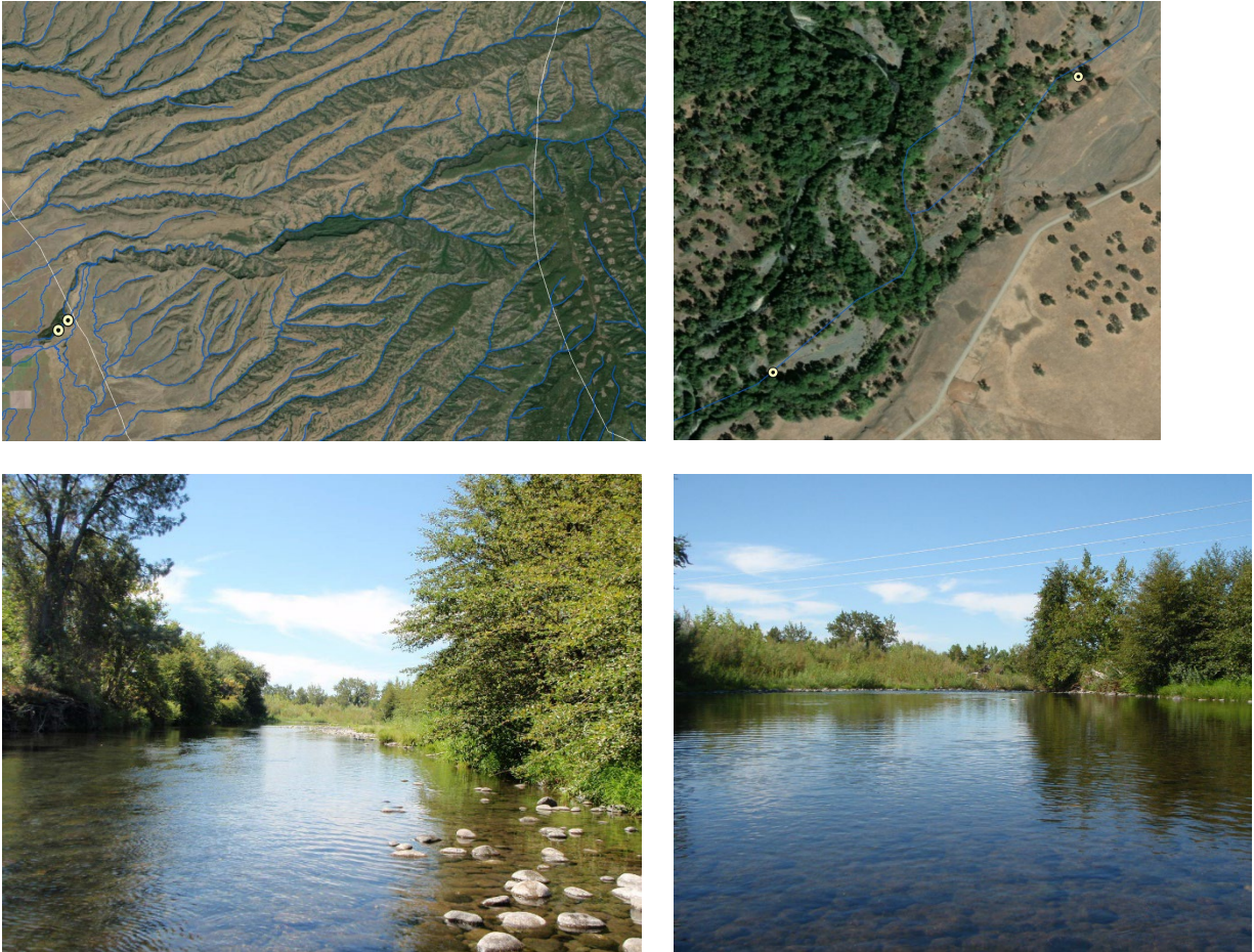
Figure 8. Aerial imagery (top row) and field photos (bottom row) of Deer Creek, reach on the Central Valley floor site with CSCI scores above 0.9.
