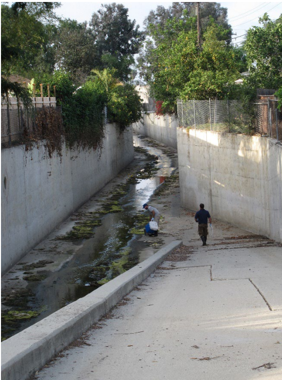
Figure 30. Examples of reaches with hardened streambeds. Left: Fullerton Creek (Orange County) has hardened bed and banks. Right: Morrison Creek (Sacramento County) has a concrete-lined streambed but vegetated soft sediment on the banks.
