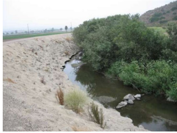
Figure 31. Examples of reaches with one hardened bank. Left: The Arroyo Seco (Los Angeles County). Right: Conejo Creek (Ventura County).
