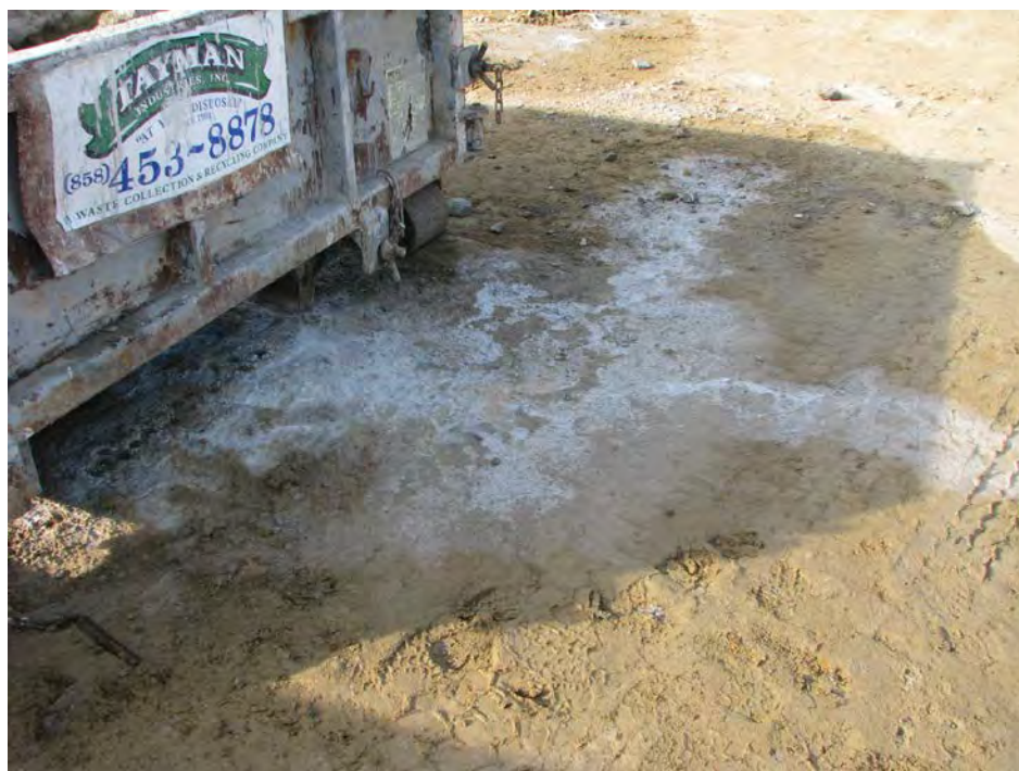
Figure 8. Concrete staining on soil from leaking washouts
