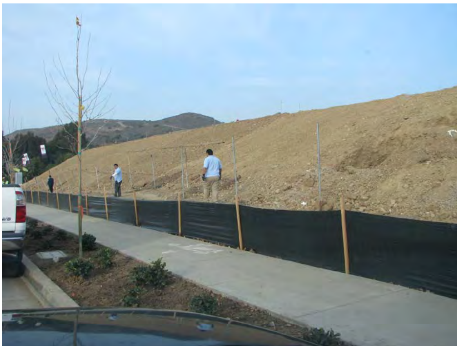
Figure 12. Slope on west side of property
