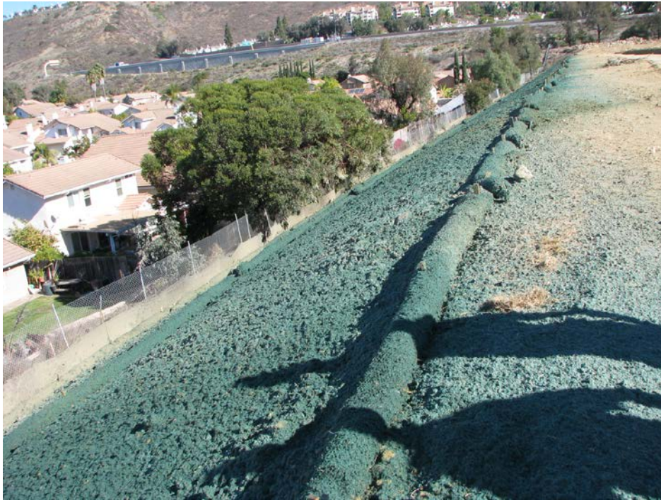
Figure 11. North slope has erosion control BMPs
