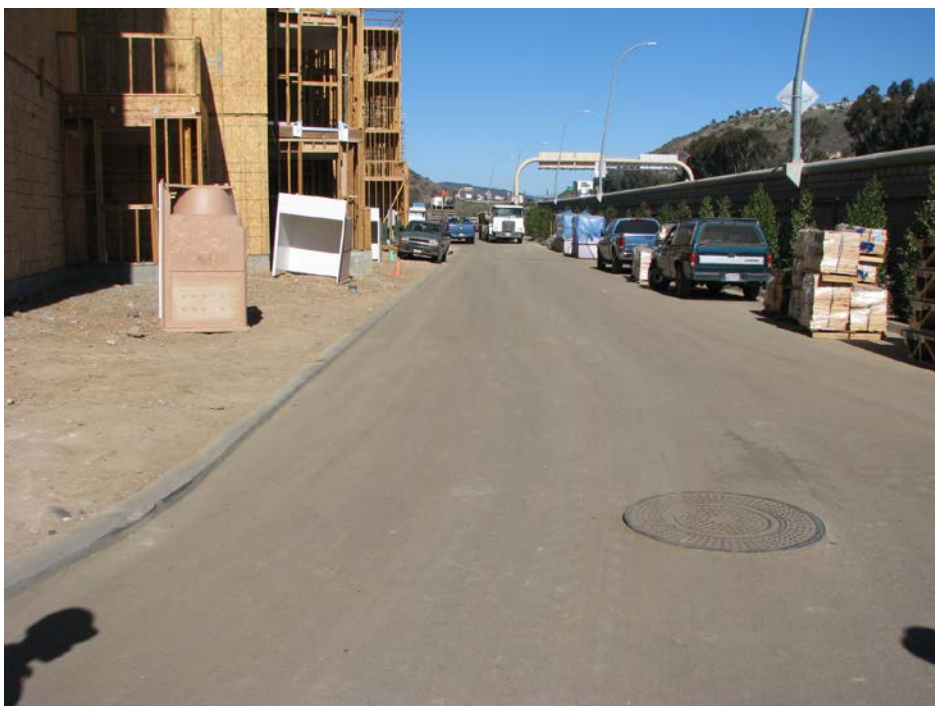
Figure 2. East side of active constructive site
