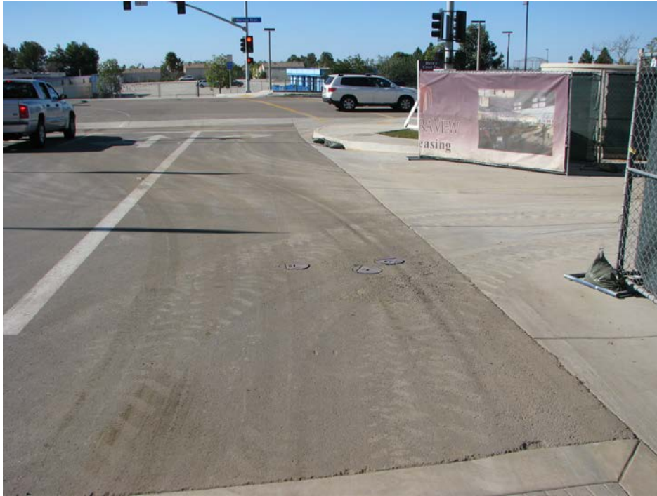
Figure 13. Construction entrance shows tracking
