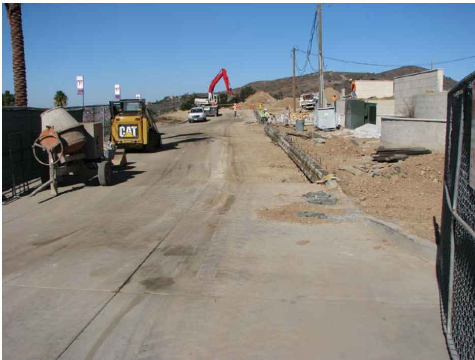
Figure 14. Looking north into construction site from entrance in Fig. 13
