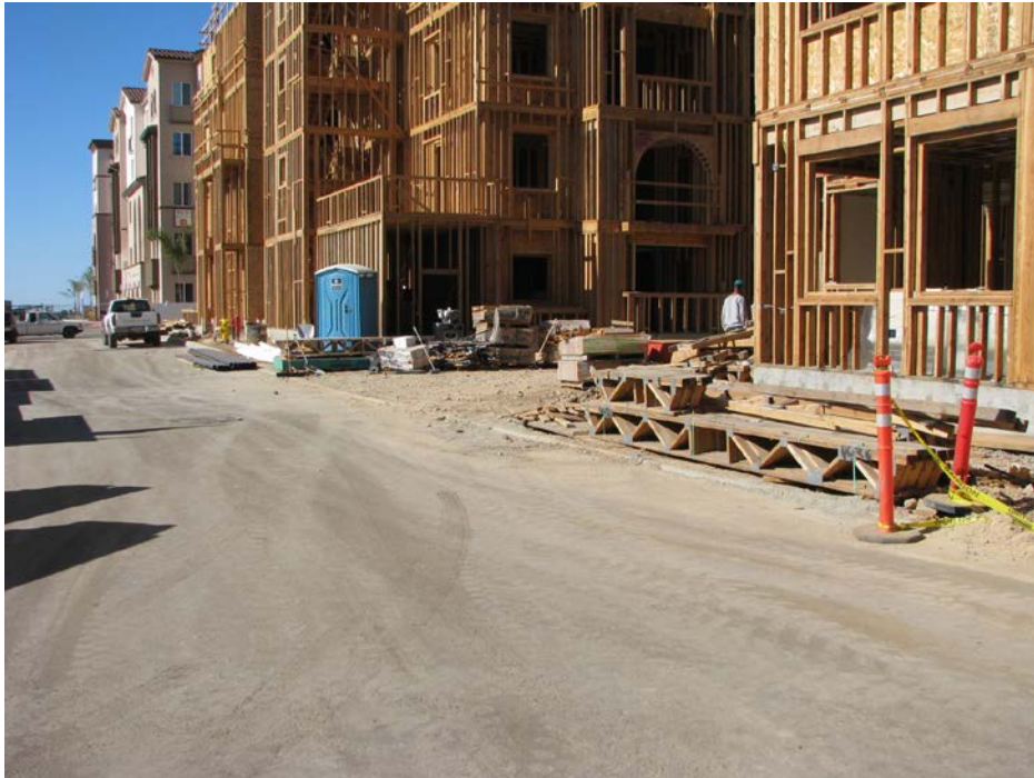
Figure 1. South side of active construction site
