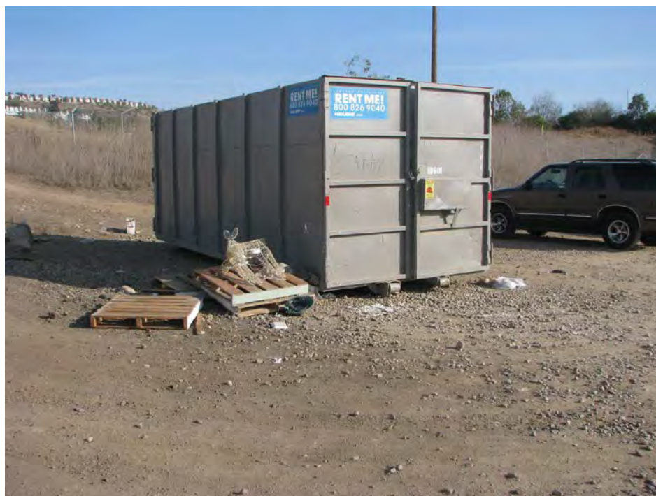
Figure 4. Site interior; construction debris
