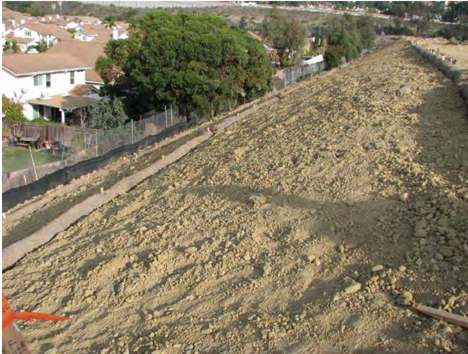
Figure 11. North slope looking easterly
