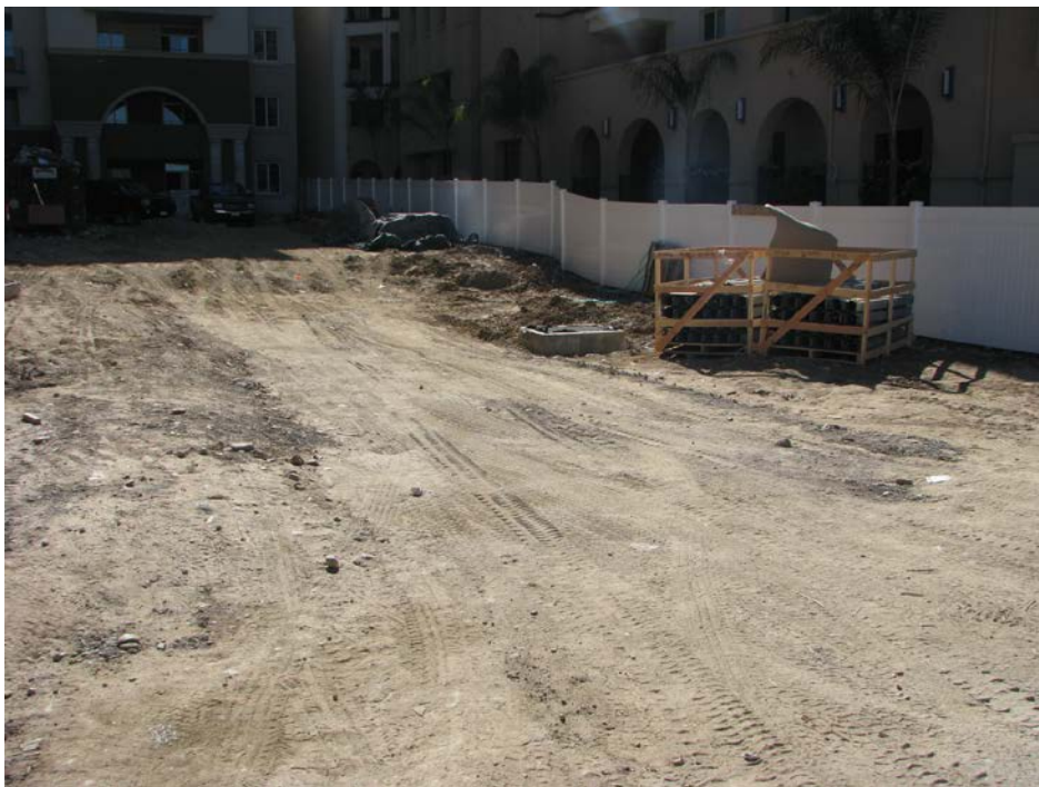
Figure 6. Site interior; trash and debris has been removed
