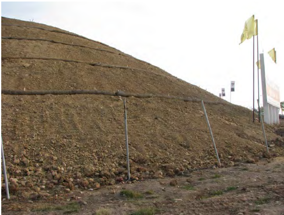
Figure 10. Slope is 2:1 Horizontal: Vertical according to SWPPP
