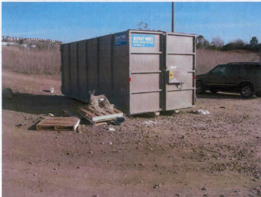
Figure 4. Site interior; construction debris
