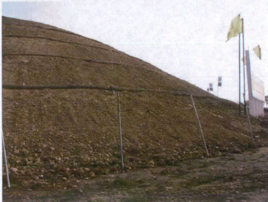
Figure 10. Slope is 2:1 Horizontal: Vertical according to SWPPP
