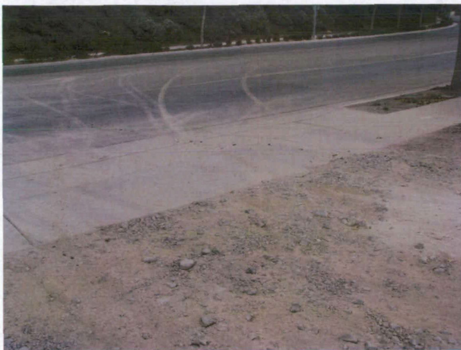
Figure 17. Gravel at south entrance
