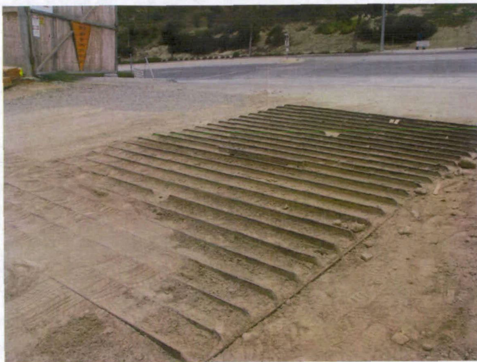
Figure 15. Shaker plates north entrance
