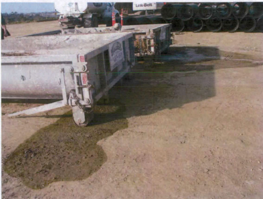
Figure 7. Leaking concrete washouts
