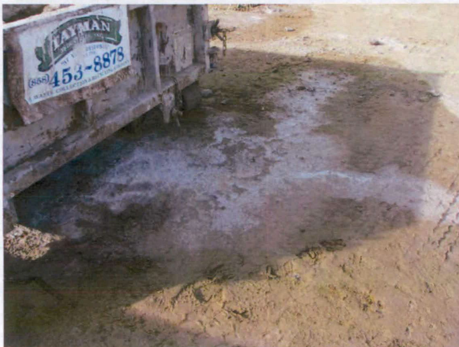
Figure 8. Concrete staining on soil from leaking washouts
