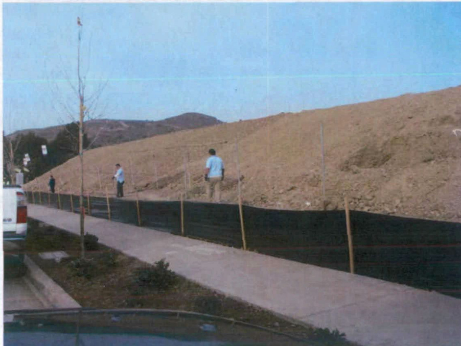
Figure 12. Slope on west side of property
