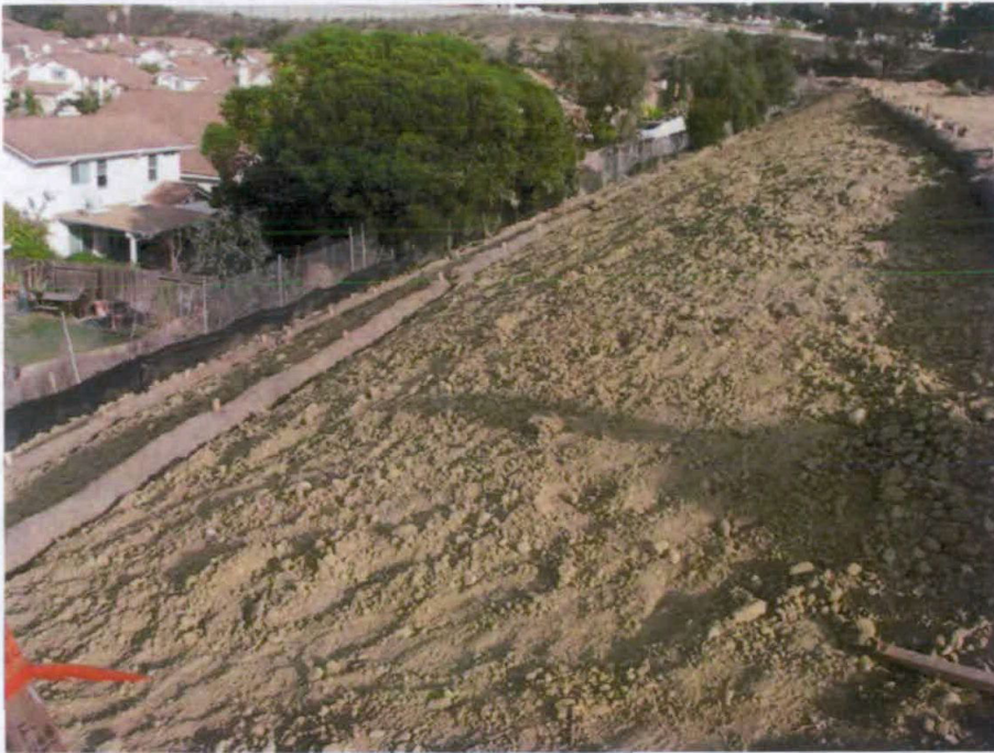
Figure 11. North slope looking easterly
