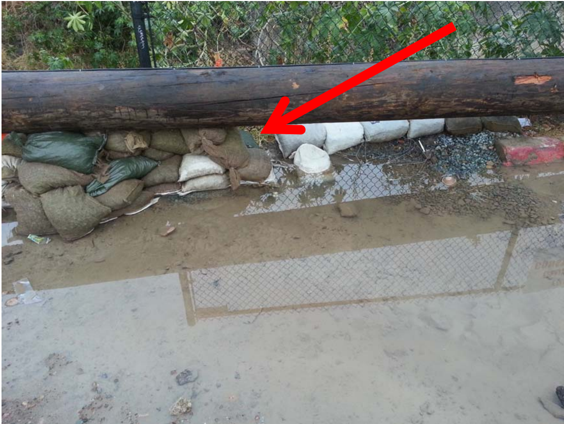
Figure 6. Failure to implement perimeter sediment control BMPs. Photograph taken by Frank Melbourn, San Diego Water Board on May 8, 2015, of gap (identified by red arrow) in perimeter sediment control BMPs that resulted in sediment discharge to Encanto Channel. 20150508_192234.jpg
