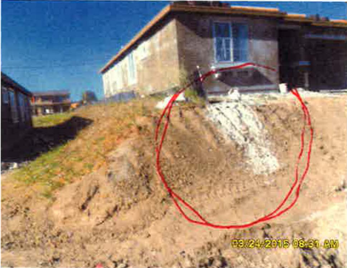
Figure 13. Failure to prevent the discharge of concrete waste to the ground. Photograph taken by the City of Lemon Grove on March 24, 2015, depicting discharge of concrete waste on slope (identified by red circle).
