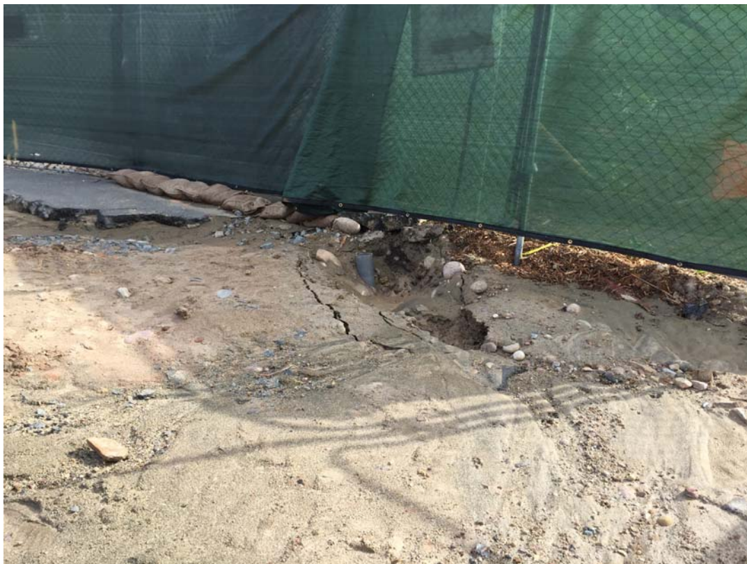
Figure 9. Failure to manage run-on and runoff. Photograph taken by Wayne Chiu, San Diego Water Board on December 15, 2014, displaying erosion caused by runoff flowing under fence and offsite. IMG_5042.jpg.
