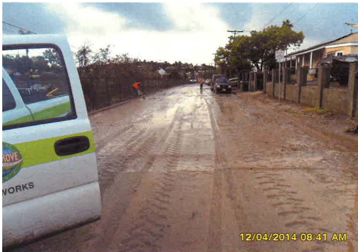
Figure 10. Failure to remove sediment from roads. Photograph taken by the City of Lemon Grove on December 4, 2014, depicting sediment on Akins Avenue southwest of the Site.
