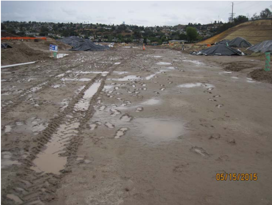
Figure 7. Lack of erosion control BMPs in active areas. Photograph on May 15, 2015, of muddy thoroughfare (Tangelos Place) lacking erosion control BMPs after rain event. Photograph taken by Frank Melbourn, San Diego Water Board. IMG_0354.jpg
