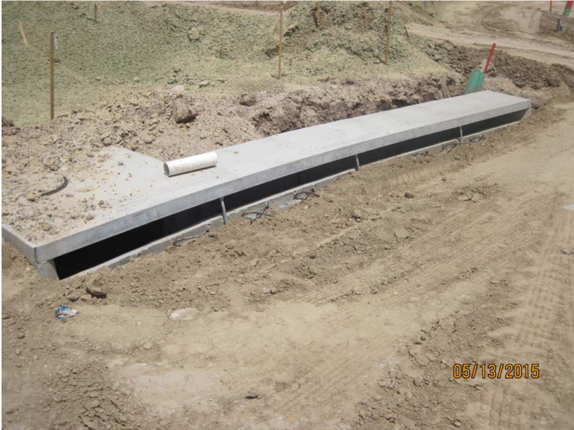
Figure 11. Failure to protect storm drain inlets. Photograph taken by Frank Melbourn, San Diego Water Board on May 13, 2015, displaying unprotected storm drain inlet. IMG_0295.jpg.
