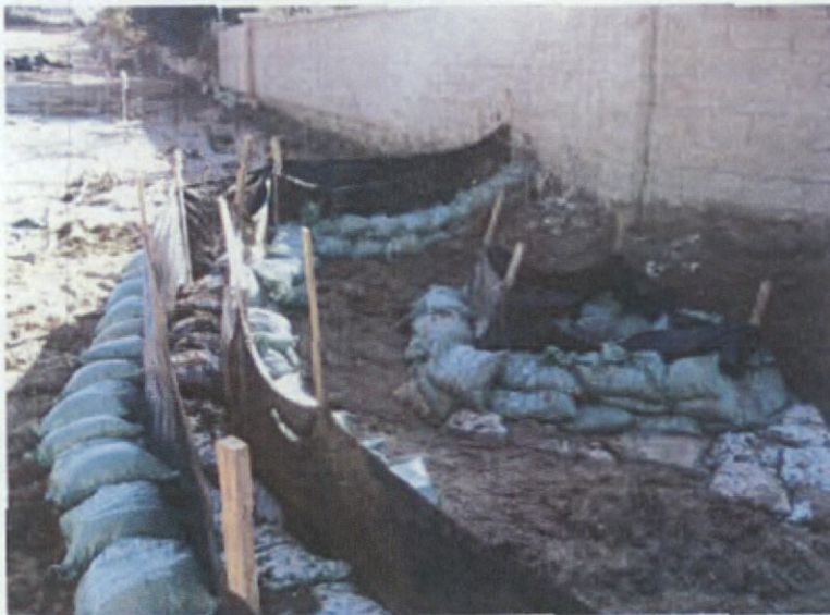
Photo 7: Inundated storm drain inlet. Green gravel bags and two outer silt fences were installed after the December 13, 2012 discharges.
