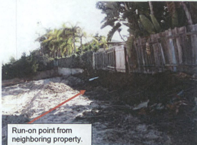
Photo 3: Lack of run-on protection from slope drain from neighboring residence that discharged to dog park area.
