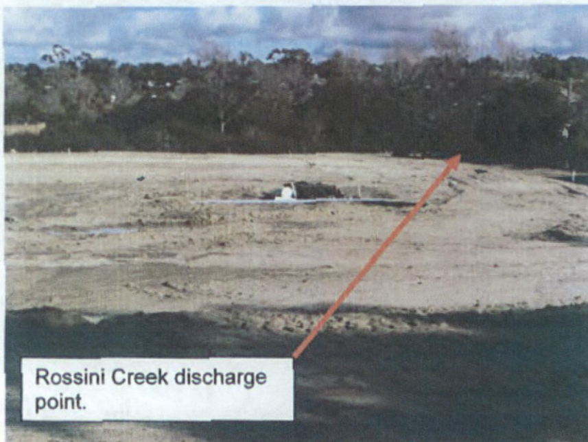
Photo 2: Dog park area located along Santa Fe Drive tributary to Rossini Creek with no erosion control BMPs.
