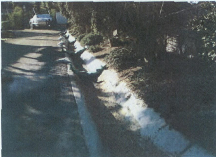
Photo 6: Sediment discharged to MS4 from erosion in previous photo.
