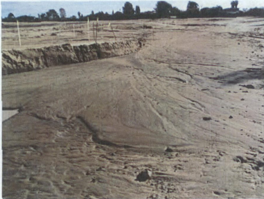
Photo 1: Large graded area with no erosion or sediment controls. Looking south towards Caretta Way.
