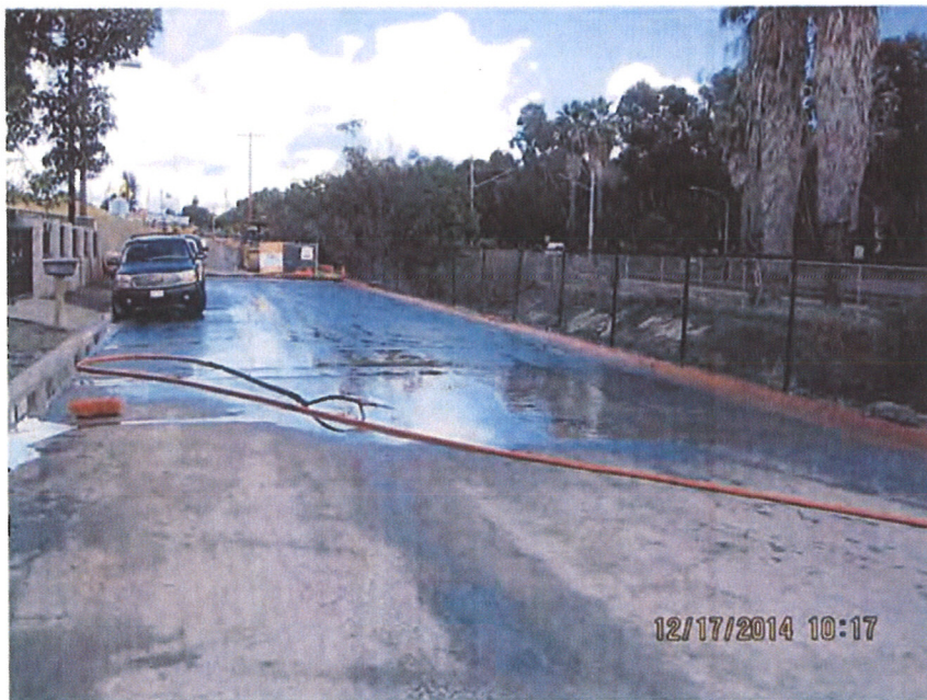
Photo 4. Power washing activity performed by Downstream Services
