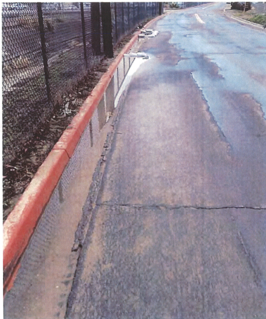
Photo 5. Sediment Accumulation along Akins Avenue, Close to Inlet
