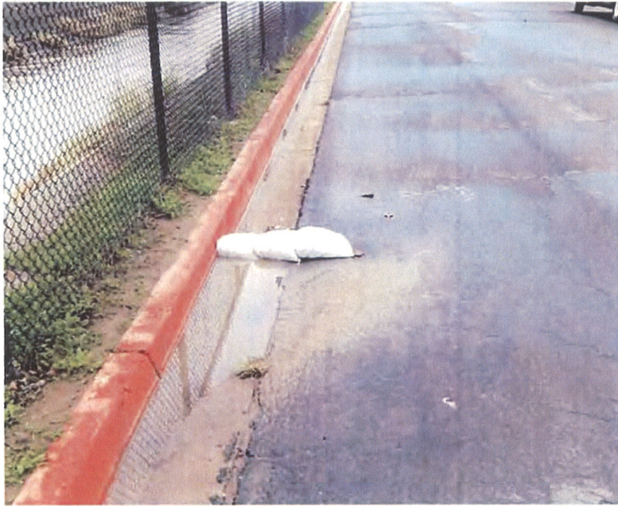
Photo 4. Evidence of Discharge Carrying Sediment around Gravel Bags along Akins Avenue
