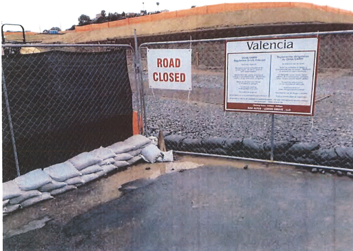
Photo 1. Ponded Water at Akens Avenue Entrance/Exit
