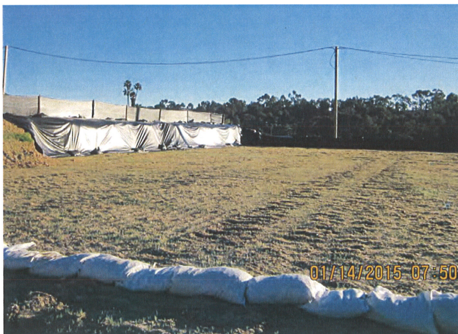
Photo 6 Sidewall protected with plastic sheeting.
