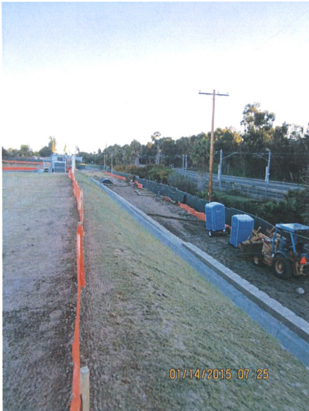
Photo 4. Rills filled in, area re-hydroseeded, silt fence added to perimeter of lot.
