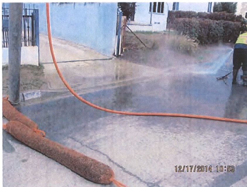
Photo 6. Power washing activity performed by Downstream Services
