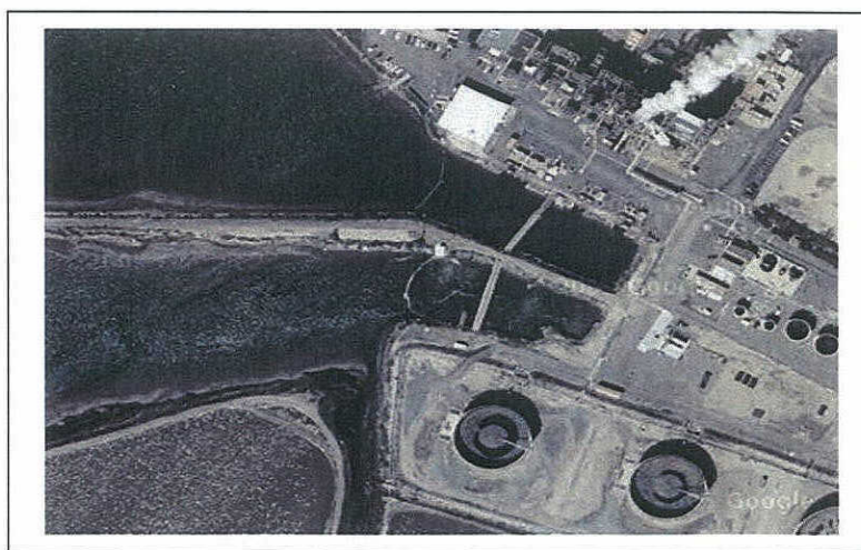
Figure 2-3. Aerial view of SBPP intake and discharge bays.
