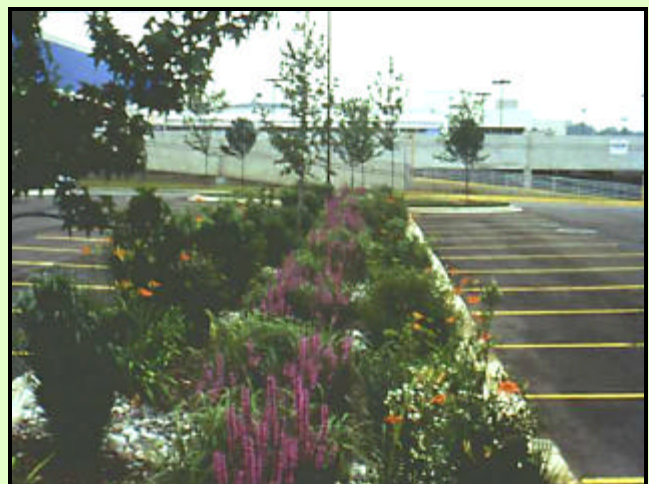
Figure 1. Bioretention landscaping at the Inglewood demonstration project site.
