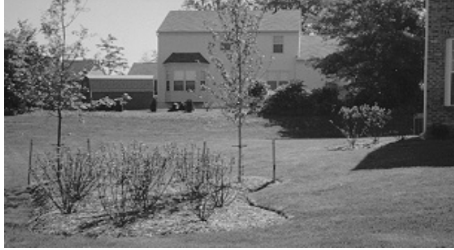
INDIVIDUAL BIORETENTION AREA
