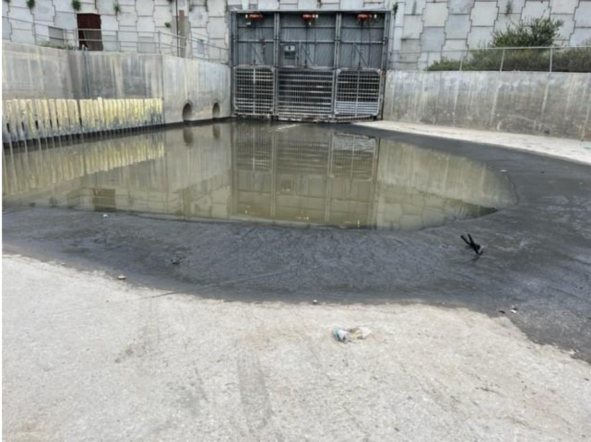
Figure 3: Goat Canyon Collector Restored to Opera on 09-29-23
