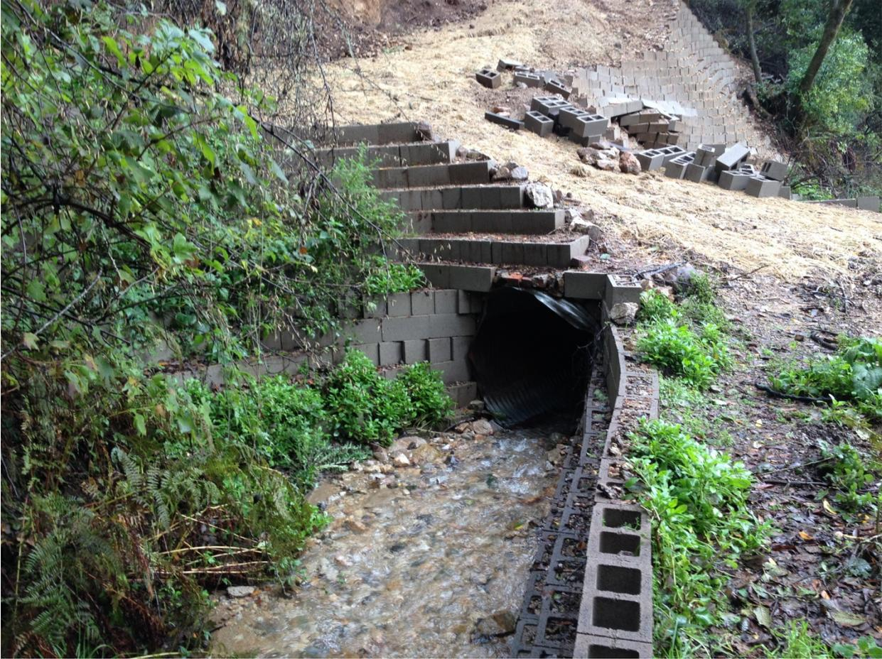
Invert of Second Unauthorized Culvert and Failing Cinder Block Wall Within and Above
