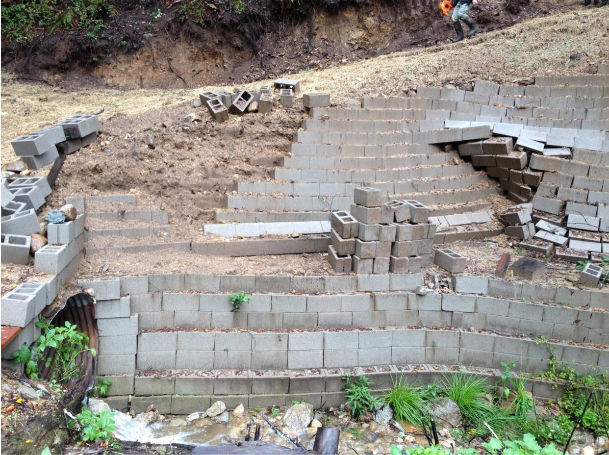
Outfall of Second Unauthorized Culvert and Failing Cinder Block Wall Within and Above Creek Bank
