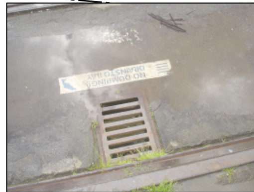
OPEN DRAIN TROUGH PIER SURFACE TO ESTUARY
