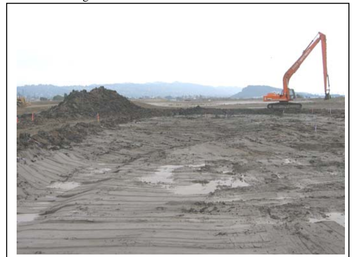
Figure 2. Same area in November 2003 after removal of debris and partial remediation.
