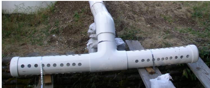
Figure 1: Perforated discharge piping
