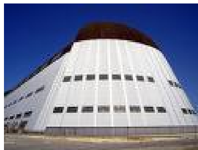
Hangar 1 exterior, doors closed
