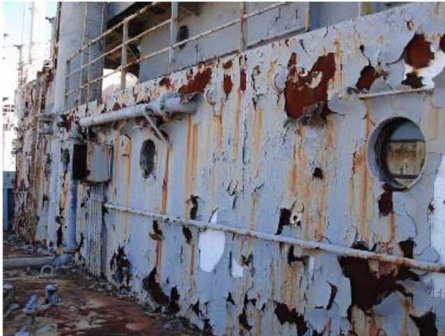
Photo #4 – Example of major paint exfoliation of an inboard surface
