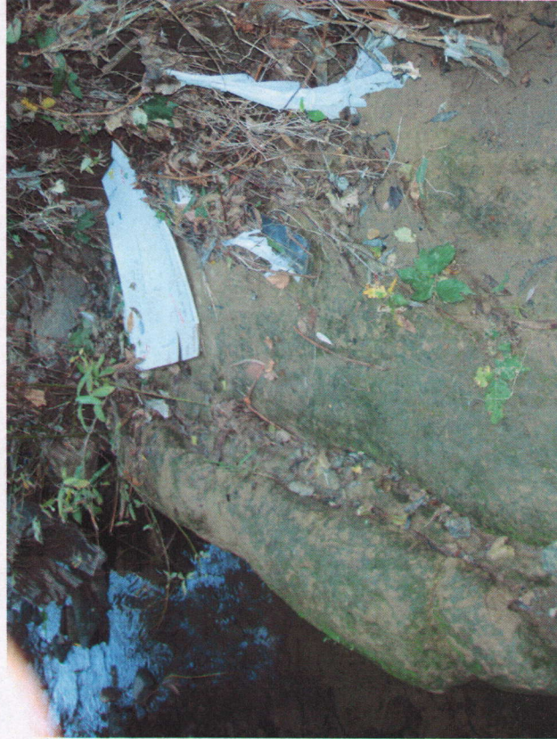
Sub optimal conditions and accumulations at catch point.
