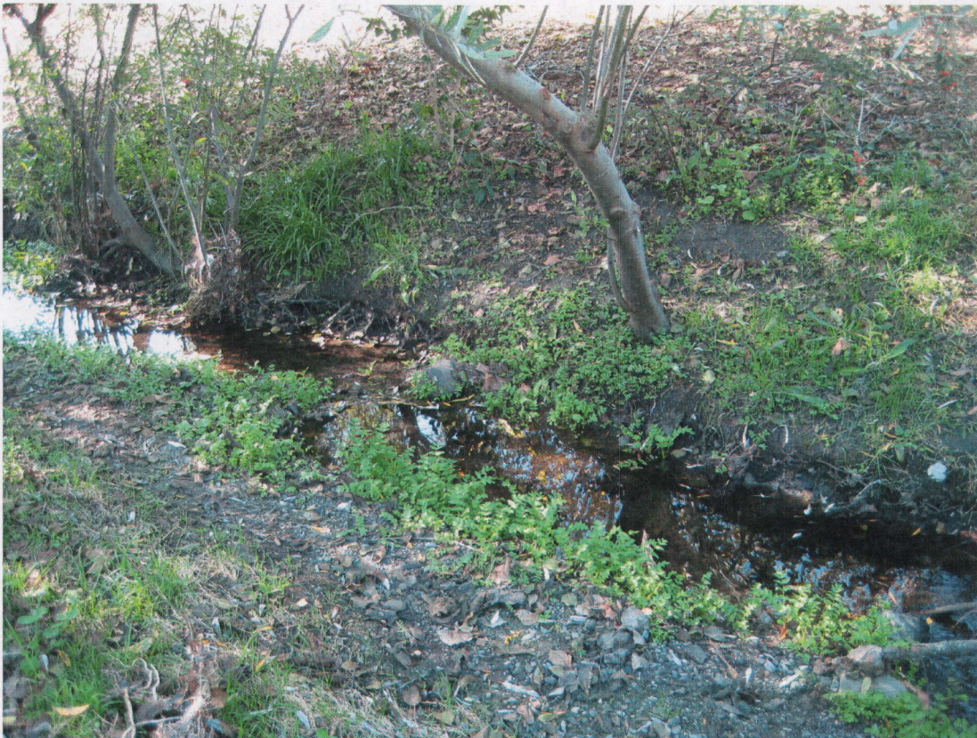
Booker T Anderson 12 4 08, downstream of bridge, stormwater 001
