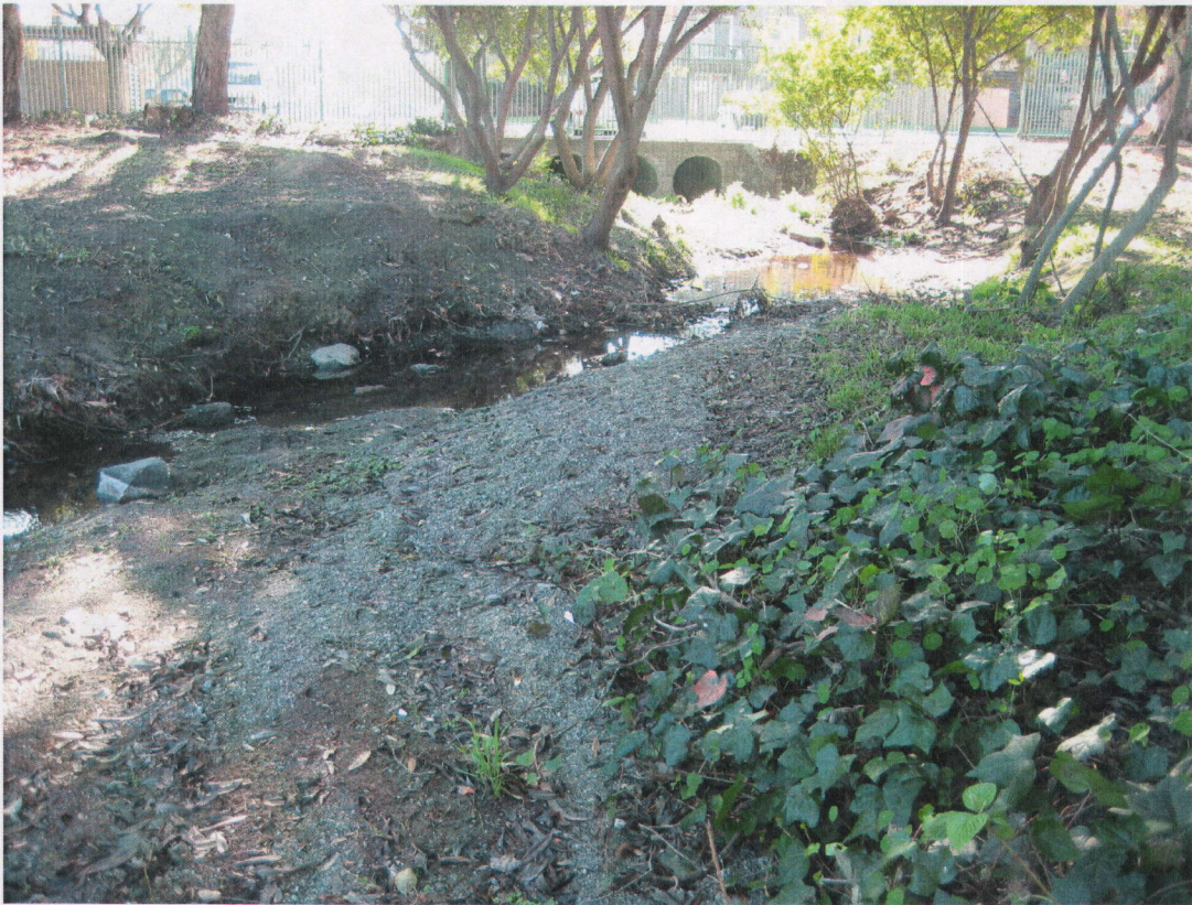
Booker T Anderson 12 4 08, bottom reach closest to housing, stormwater 003
