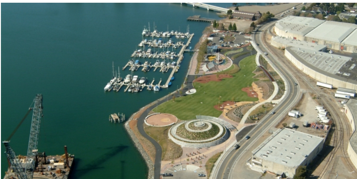
Figure 1a. Oblique northwest view from aerial photograph of Union Point Park. Contaminated soil is contained beneath the mound in the foreground with the spiral pathway and beneath the parking lots. Source: Center for Creative Land Recycling.
