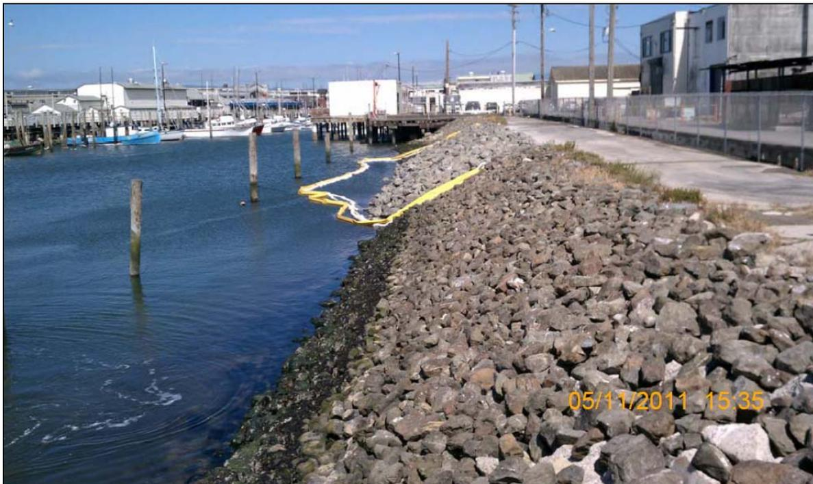
Figure 2. The Shoreline is Restored after the Removal of Contaminated Sediments.
