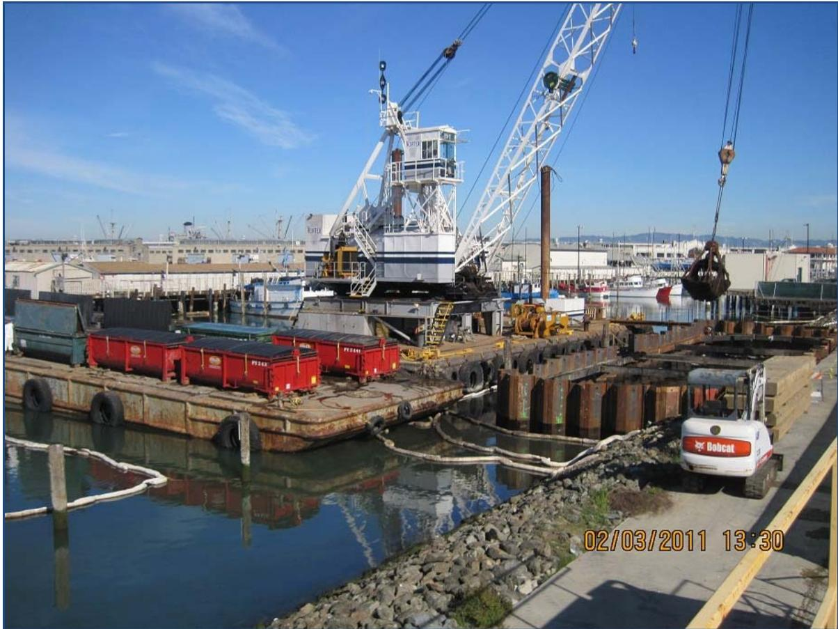
Figure 1. Contaminated sediments removed from sheet pile area and placed in red containers for offsite disposal.
