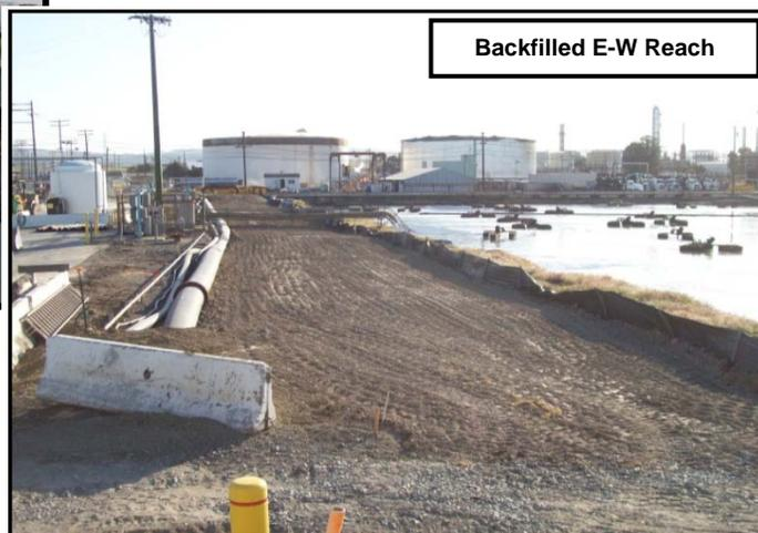
The Golden Eagle Refinery removed the oily sediments and backfilled the canal with clean rock and soil. The Refinery employed both mechanical excavation and hydraulic vacuum methods to remove the oily waste and disposed of approximately 10,000 tons of waste offsite.
