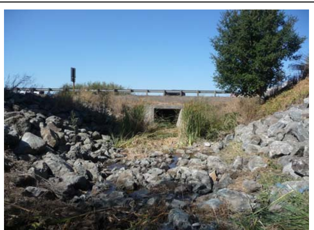
(4) Recent bank stabilization work performed by District included riprap placement upstream of the Highway 29 culvert crossing (view is looking downstream, September 22, 2010).
