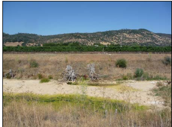
(2) In the upstream portion of the reach, the channel has a trapezoidal cross-section with minimal riparian habitat. A thick layer of algae covers the channel bed. Vegetation along the banks is primarily non-native, invasive herbaceous species and eucalyptus. (Looking east from the west bank, August 4, 2010).
