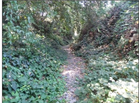
(2) Looking downstream near South Terrace Drive. Note the well defined low flow channel, coarse bed material and steep streambanks (September 2010).
