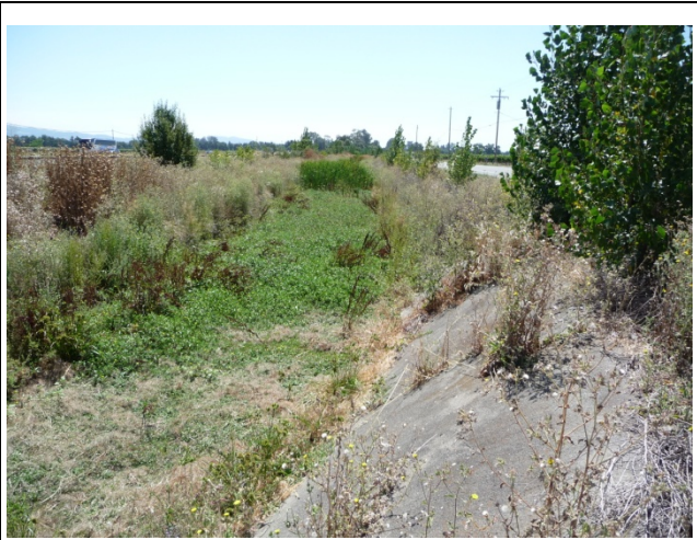
(4) Looking upstream from the confluence with the Yountville Outfall. Note dense Ludwigia in the channel (August 4, 2010).
