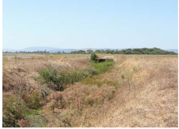
(4) In the lower portion of the reach the open channel transitions to a culverted section (background) that flows beneath the airport runways (Looking west, September 22, 2010).
