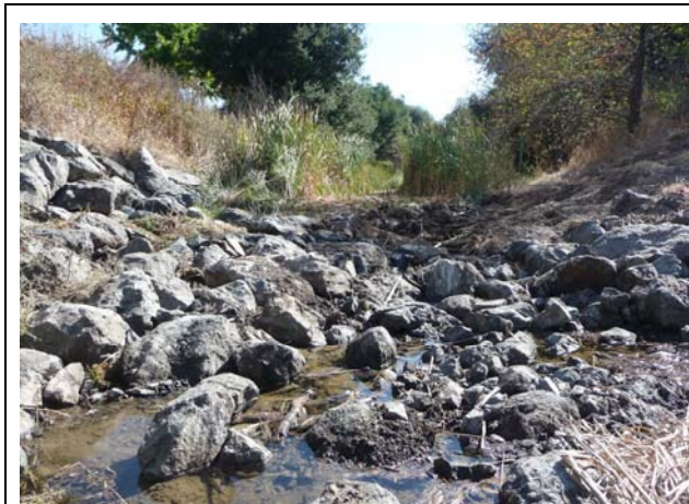
(3) Looking upstream near Highway 29 crossing. Recent riprap was placed along banks and channel bed. Channel bed and riprap crossing create depositional area upstream where sediment accumulates and cattails grow (September 22, 2010).
