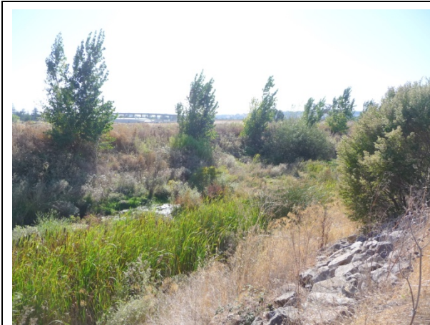
(3) Typical channel conditions near the mid-point of the reach. Note, some isolated sections of riprap are found along the banks (Looking downstream, September 22, 2010).
