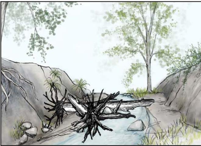
Photo 3. Downed tree, cut into smaller sections and repositioned in the channel to create in-stream complexity.
