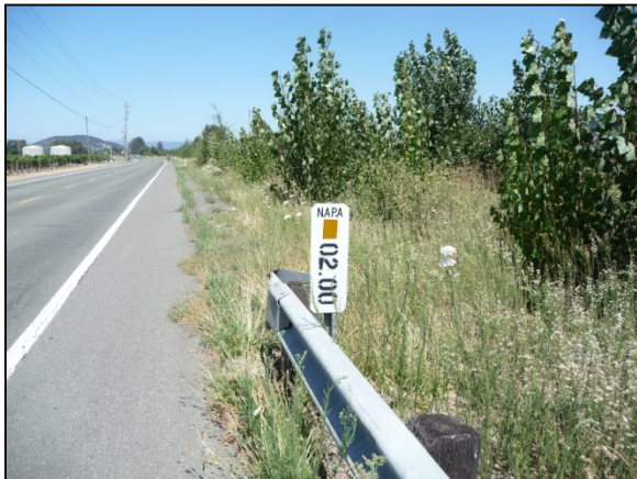
(1) Upstream end of the SYC- Reach 2. The culvert at Mile Marker 2.0 marks the upstream end of the reach. Note the cottonwoods planted along the channel ( Looking downstream, August 4, 2010 ).
