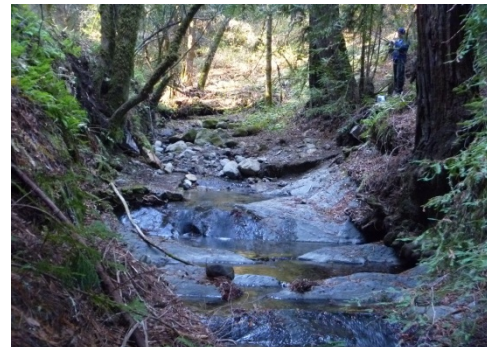
Wing Canyon Creek after removal of the abandoned instream dam in 2012
