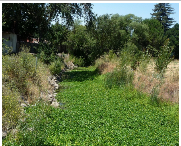
(4) Looking upstream from Jefferson St. Note riprap at the toe of slope on south bank (left side of photo) (July 2010).
