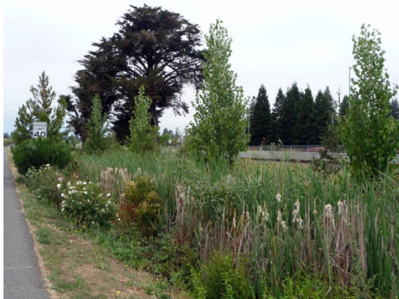
(1). Typical section of the SSC (Looking downstream from upper portion of the reach; August 4, 2010). Note dense emergent vegetation growing in the channel.
