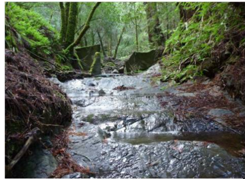
Abandoned instream dam on Wing Canyon Creek before removal
