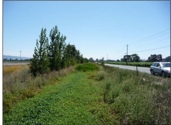
(2) Looking downstream near Vineyard View Drive. The channel supports interspersed patches of aquatic vegetation dominated by Ludwigia (foreground) and emergent vegetation dominated by broad-leaved cattail (background). Note cottonwoods planted by District on east (left) bank (August 4, 2010).
