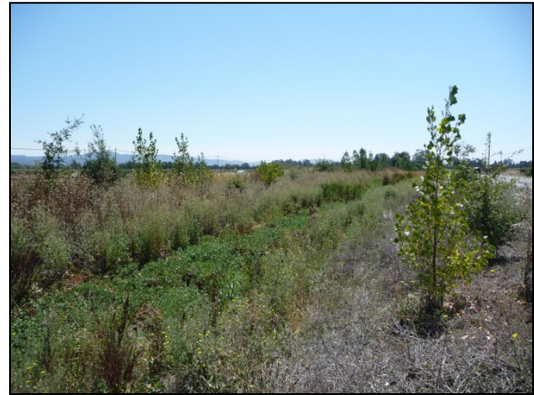
(2) Looking upstream in the mid-portion of SYC Reach 2. The channel is formed in native soils. Dense aquatic vegetation, such as Ludwigia , grows in the channel ( August 4, 2010 ).
