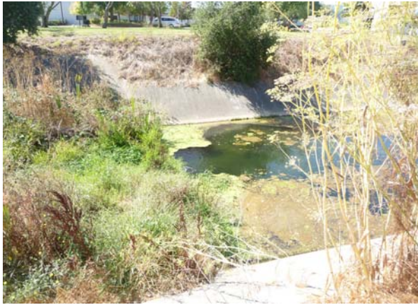
(3) A sediment “plug” has accumulated upstream of a concrete-reinforced cross-section of the channel. (Looking west, September 2010).
