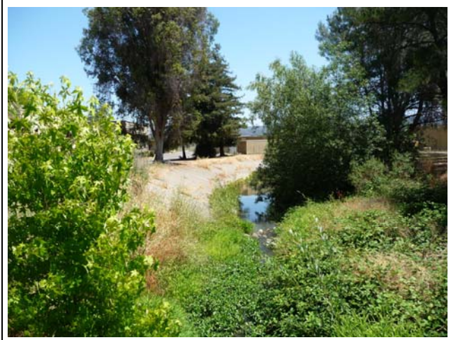
(4) Looking downstream from a bridge in the lower portion of the reach. Note concrete lining on north bank (left side of photo) (July 8, 2010).
