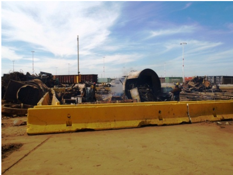
Torch-cutting station relocated to paved and contained area. Project completed – June 2012.
