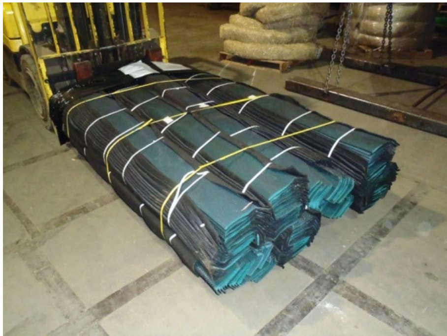
Ertec™ stormwater filtration barrier awaiting installation along edges of concrete dock. Expected project completion – October 31, 2012.
