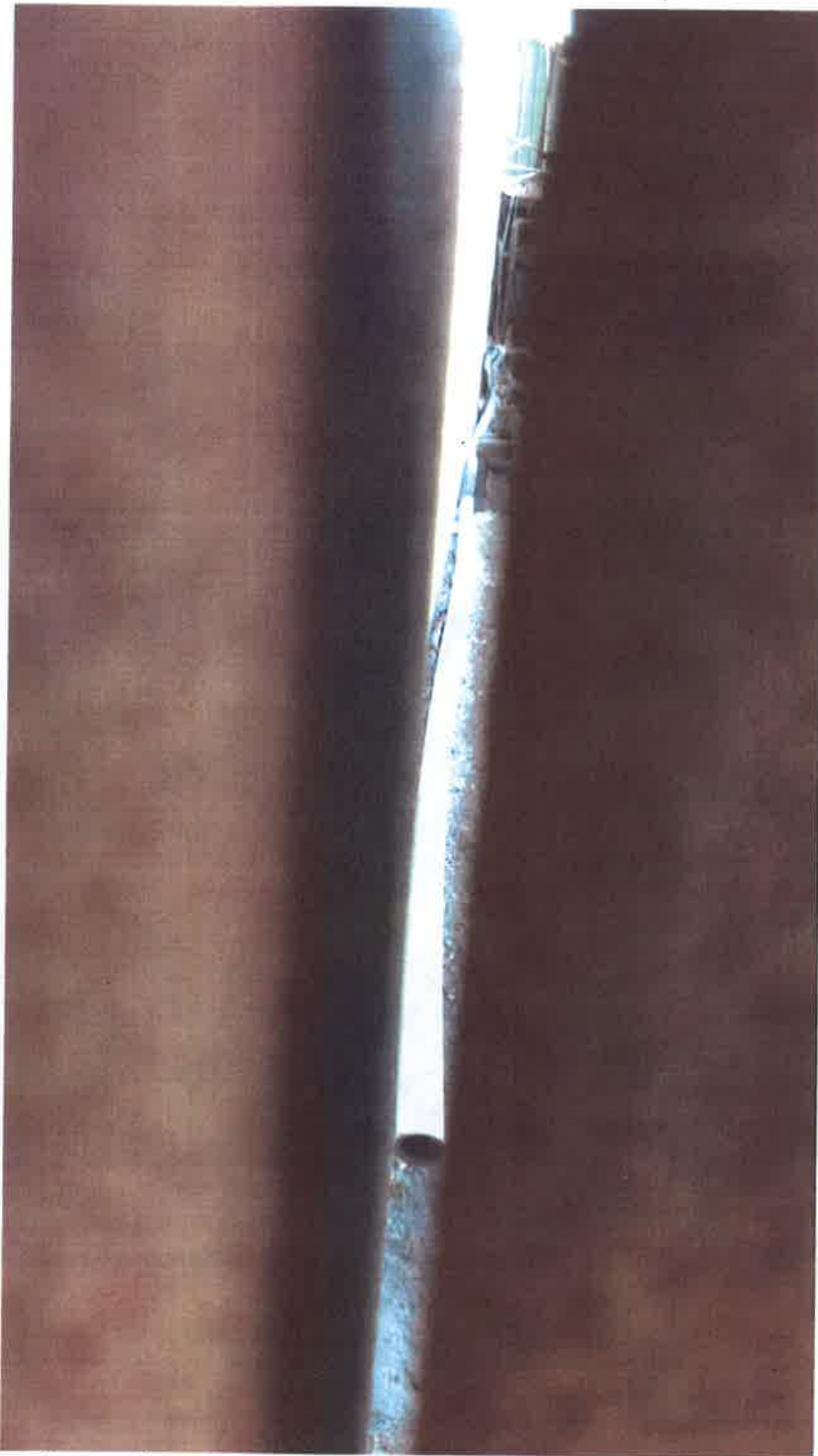
Photograph c – Pipe coming out of the E – D Coat, Inc. facility located at 715 4th Street, Oakland, California 94607. Photograph taken by David Williams on June 3, 2013, at 5:22 p.m., looking north at the back of the facility from 3rd Street.
