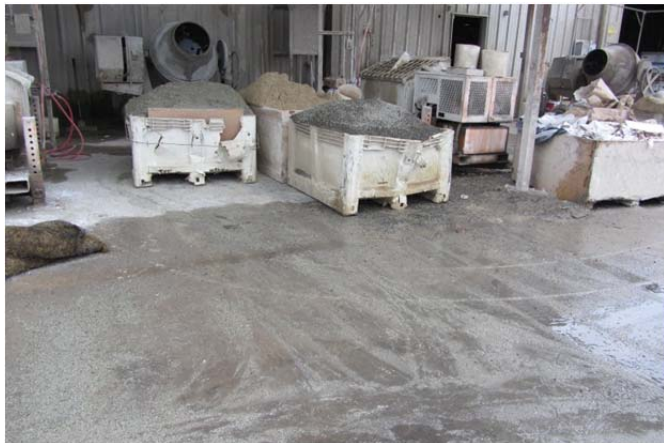
Photo O: Inadequate Industrial Material (aggregates and sand) Storage with Tracking
