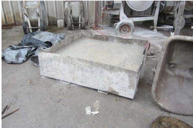
Photo R: Process Water Settlement basin without Overflow Control
