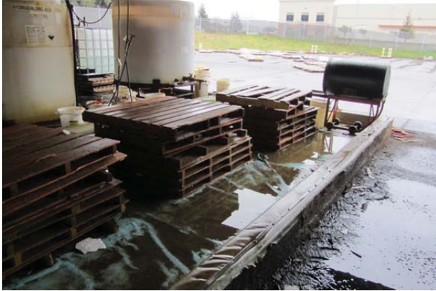
Photo A: Wastewater Treatment Area with liquid of Unknown origins in containment
