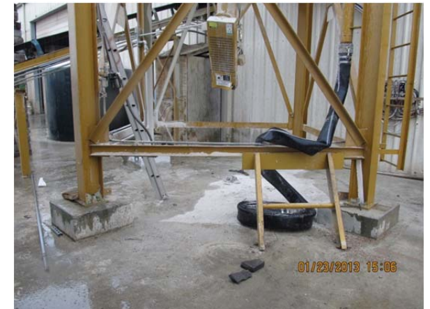
Photo Q: Aggregate Spill
