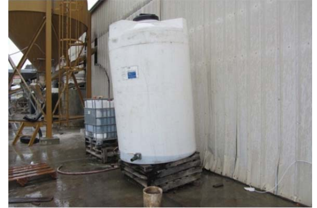
Photo H: Unsecured Outdoor Chemical (Pozzolith) Storage Without Secondary Containment
