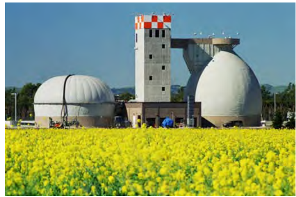
Soscol Water Recycling Facility
