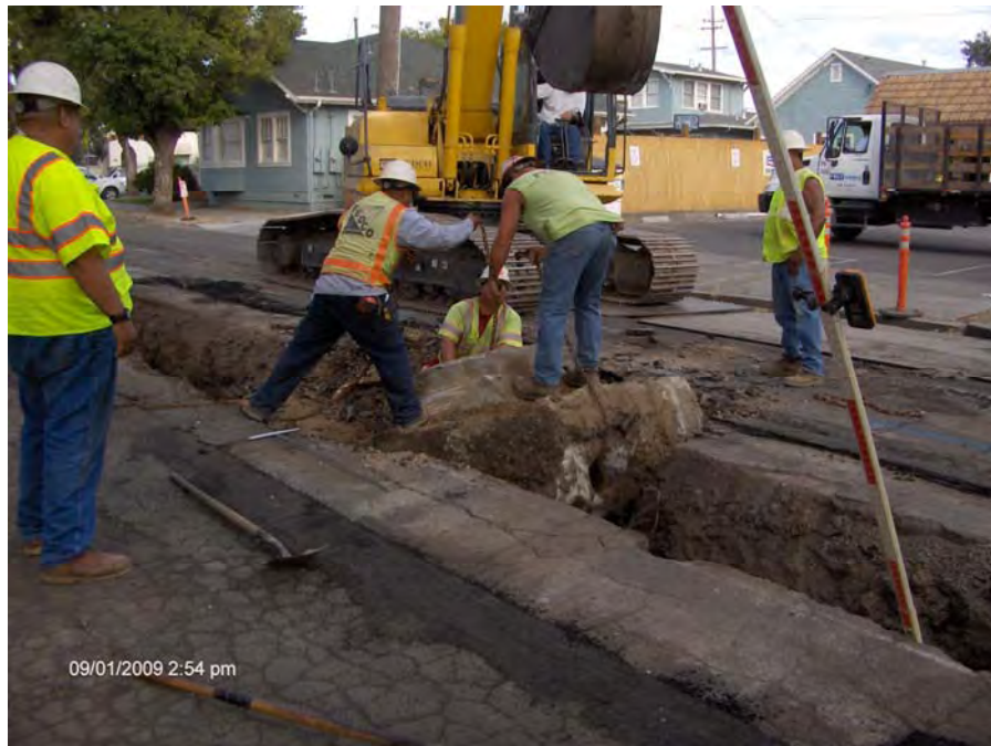
Construction during Lower Alphabet Street Sewer Improvement project
