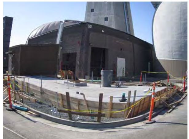
Construction of the FOG Receiving Station
