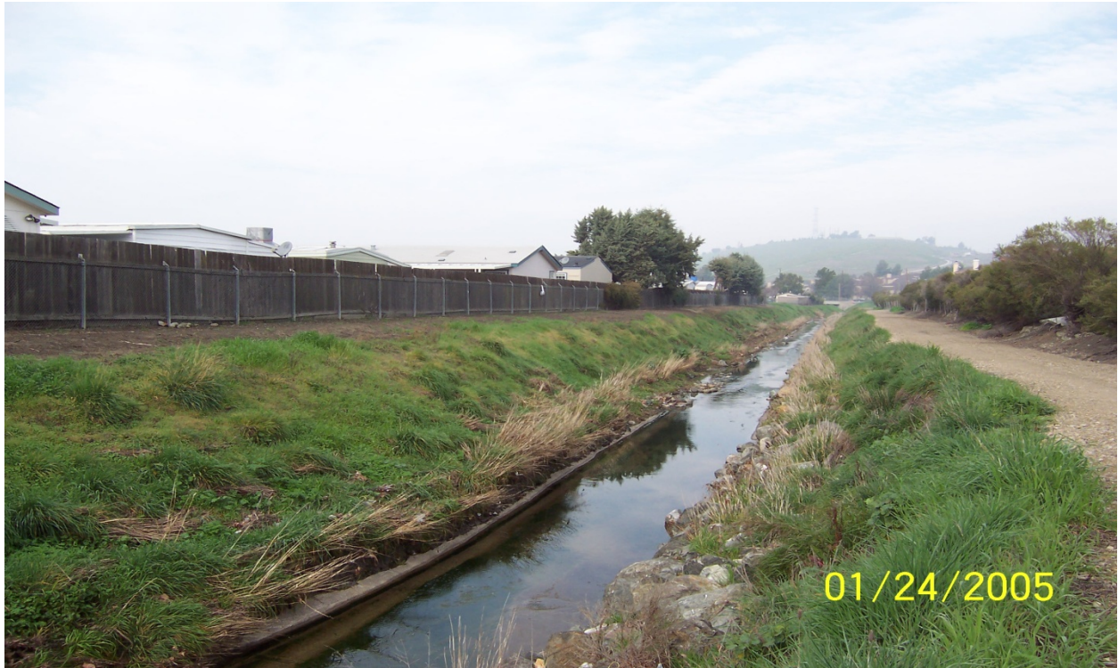
Before – Canos Creek u/s Hillsdale
