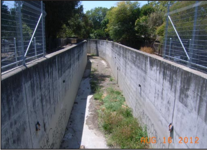
Photo 1. Adobe Creek at Station 219+16.
