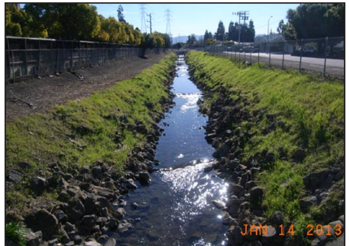
Photo 6. Sunnyvale East Channel at Station 156+28.
