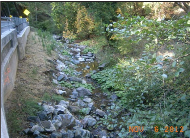
Photo 3. Stevens Creek at Station 931+46.
