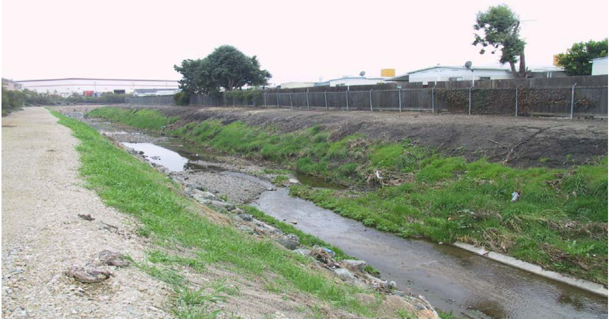
Before – Canos Creek u/s Hillsdale
