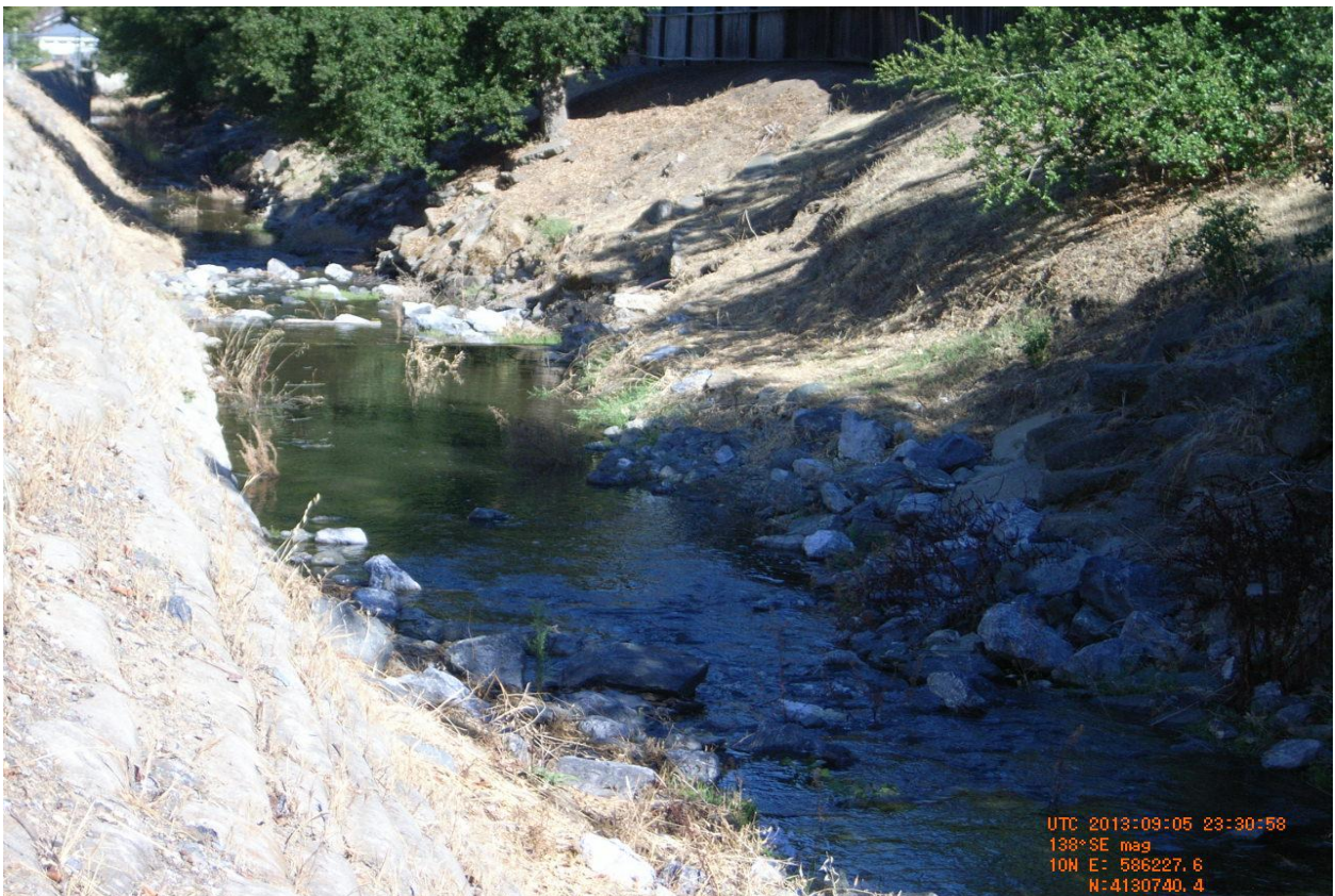
After – Regnart Creek d/s Pacifica
