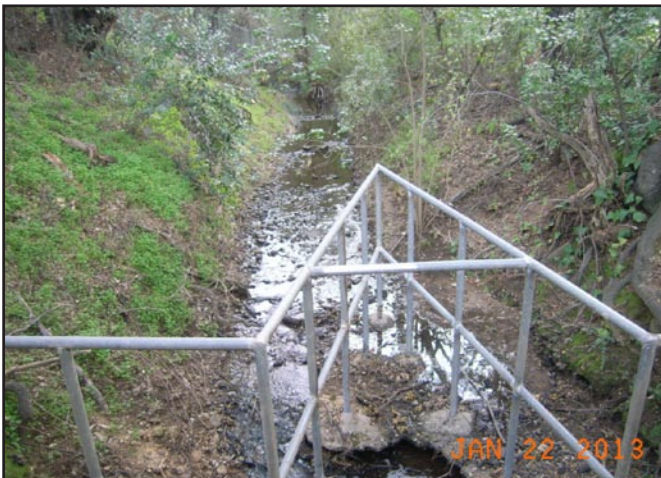
Photo 5. Smith Creek at Station 71+25.
