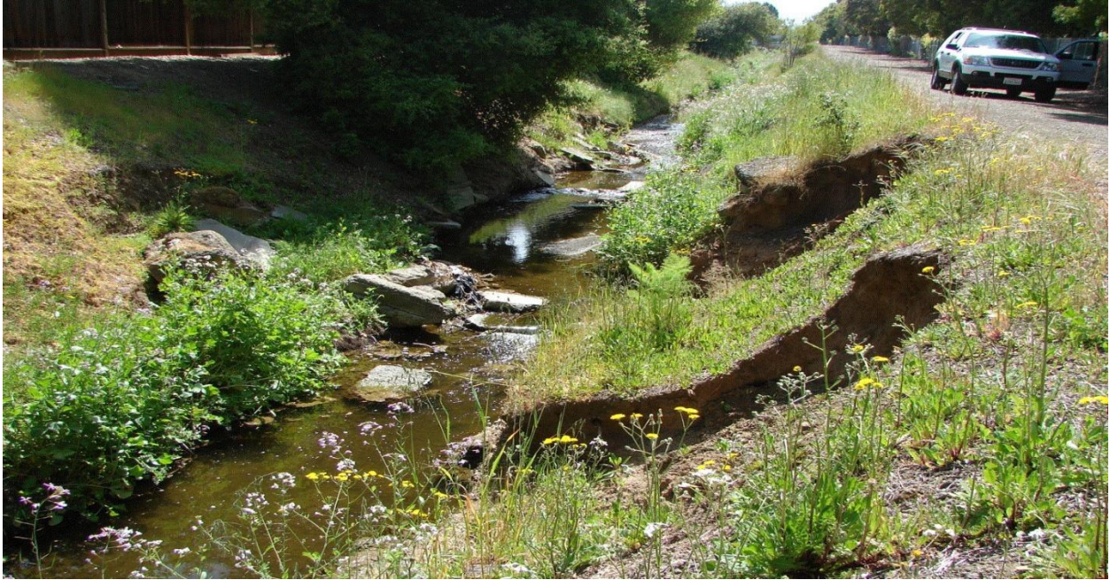
Before – Regnart Creek d/s Pacifica
