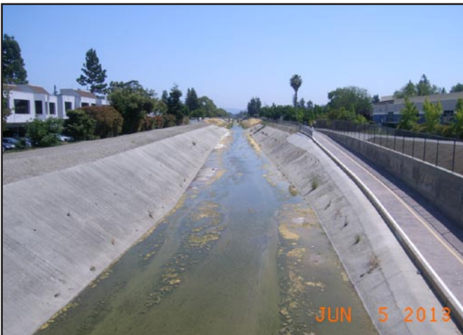
Photo 5. San Tomas Creek at Station 174+17.
