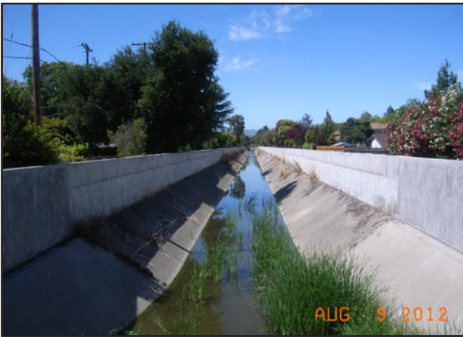
Photo 3. Matadero Creek at Station 121+08.
