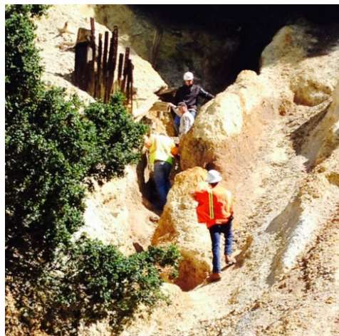
Photo 1b. Site workers inspect adit.
