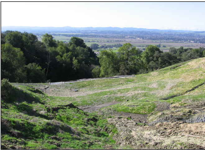
Photo c. Active slide face graded, drain pipes used to dewater surface drainage away from slide; drain, manhole cover, and detention area seen in mid-ground (Feb. 2006).
