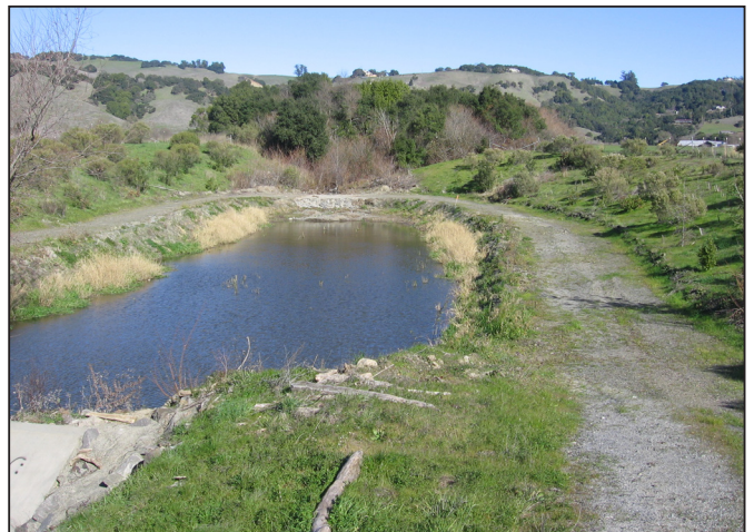
Photo f. Cook Creek Sediment Basin (July 2007), following erosion control treatments upstream, frequency and need for sediment removal at basin is diminished.
