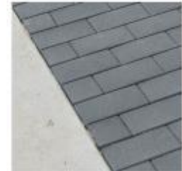
pavers with poured concrete
