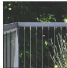
ALTERNATIVE B VERTICAL CABLE RAILING
