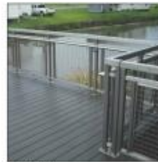
ALTERNATIVE C WIRE MESH RAILING
