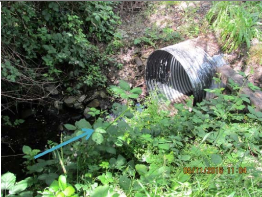
Photograph 3: Entrance of the culvert at upstream end.
