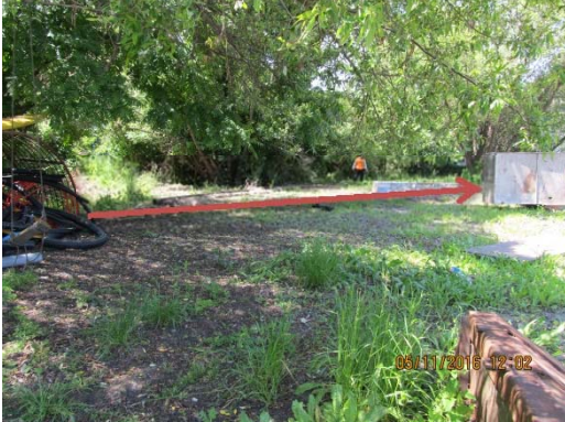
Photograph 1: Red arrow show approximate distance of culvert.
