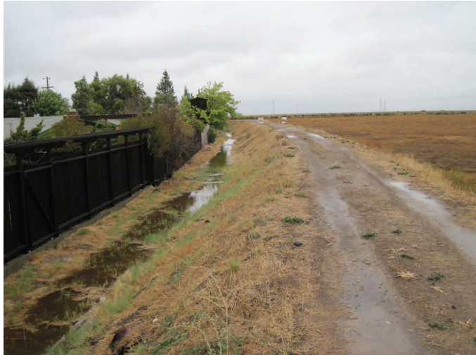
Estancia Ditch (Gallinas Creek is below levee on right).
