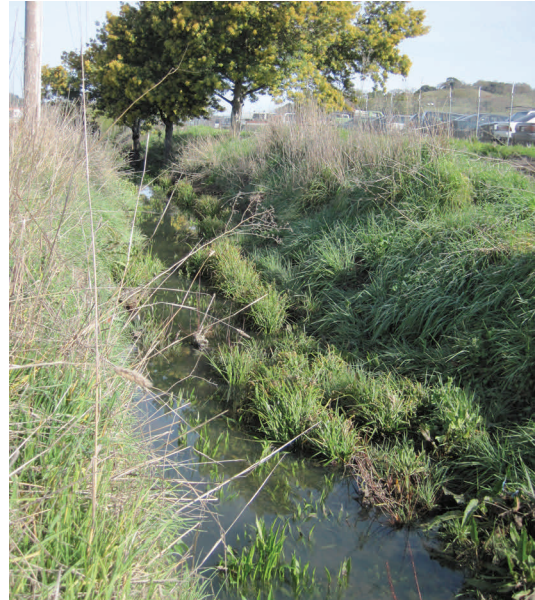
Rush Creek near Olive Ave.
