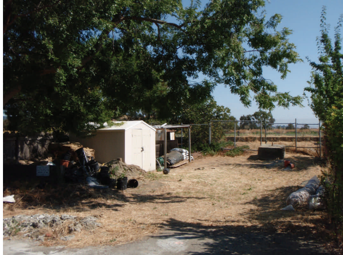
Pump station #2 between Vendola Dr and the Gallinas levee.
