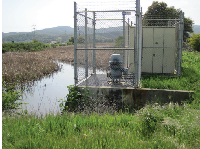
Cheda Creek pump station.
