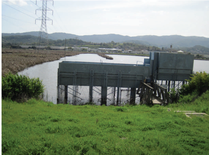
Lynwood pump station (looking west over Lynwood Slough).
