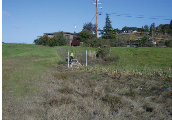
Detention basin at Pump Station #4
