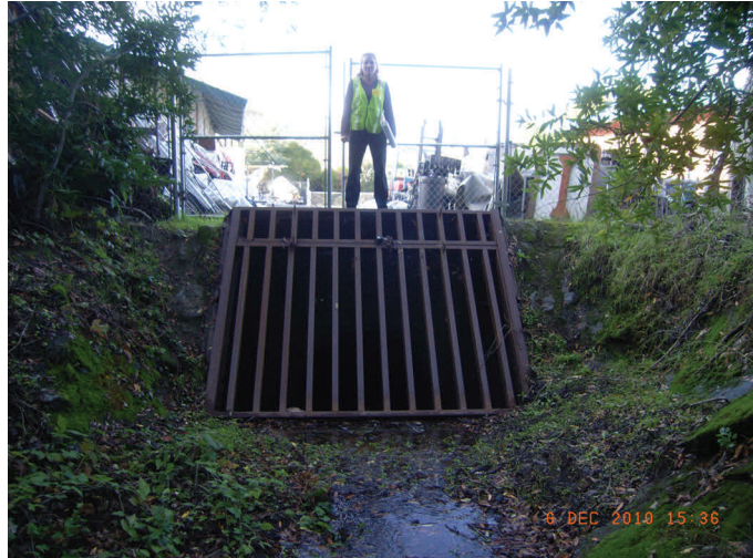
Trash rack at Meadow Way inlet, near the 7-11.
