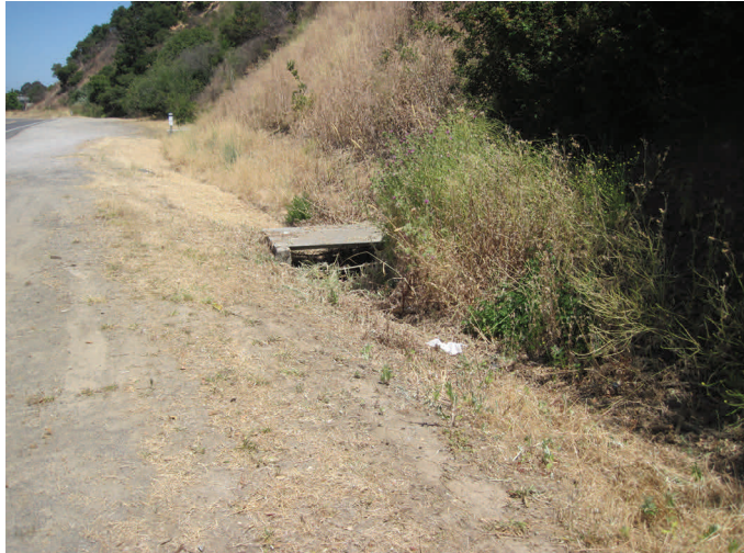
La Pasada inlet and ditch along N. San Pedro Road.
