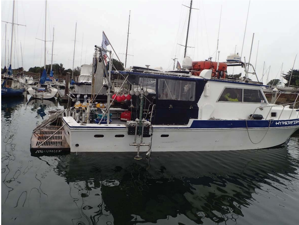
Figure 2-2. Plume mapping survey boat used for dynamic profiling for Pier E6 to Pier E18 controlled underwater blasting.
