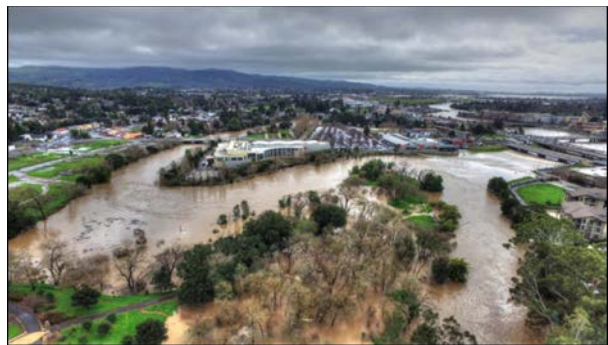
Project prevents flooding during 2017 high flows.
