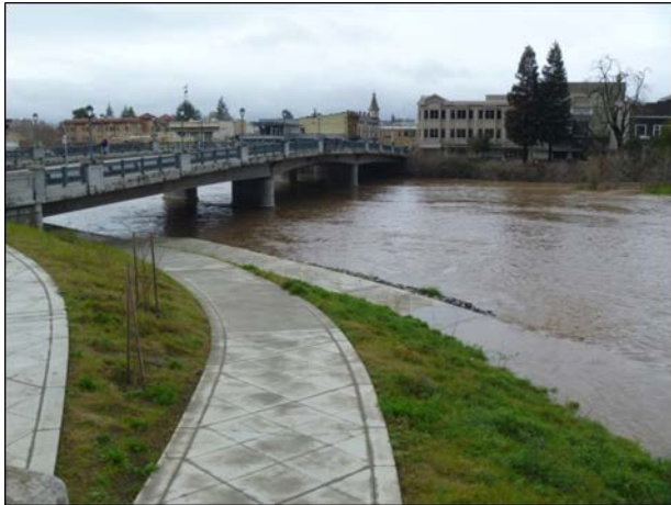
Oxbow Bypass functioning to prevent flooding.
