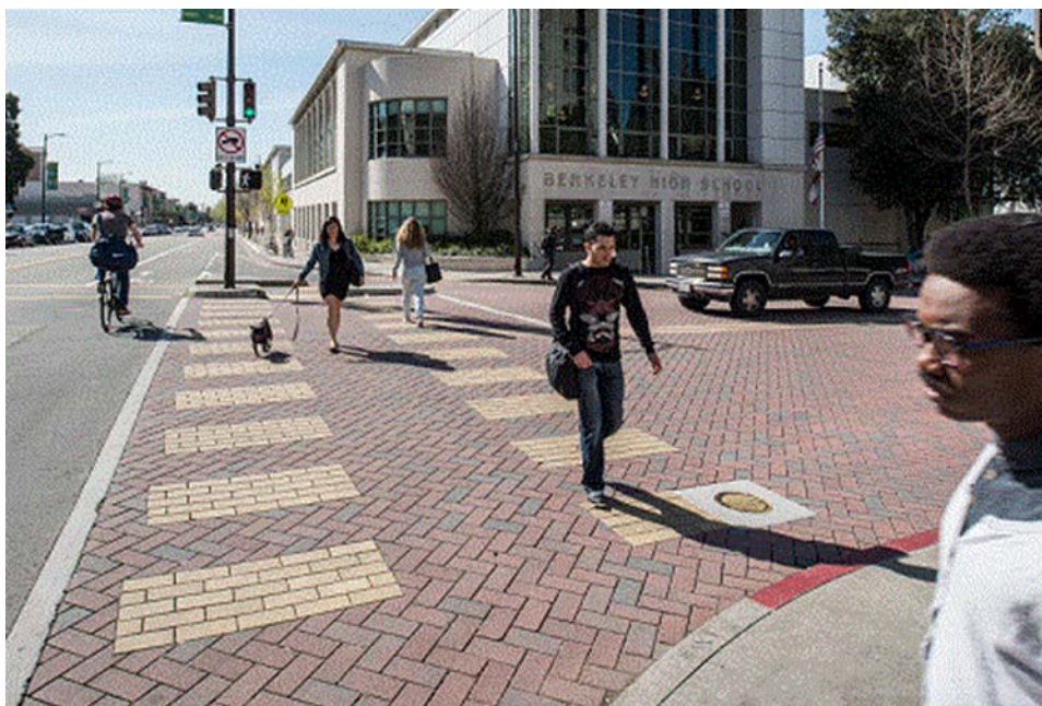
Figure 2. Permeable pavement at Allston Way, Berkeley
