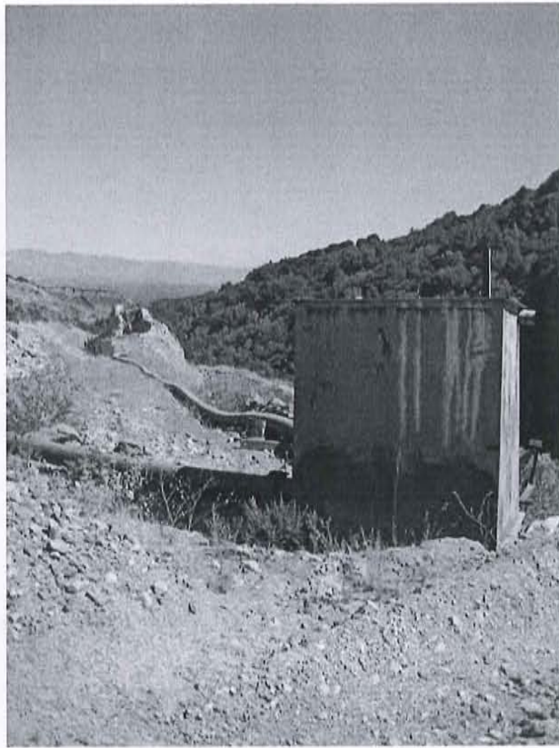
Photo 3: View of piping diverting water from the quarry pit to Pond 4 in the distance.
