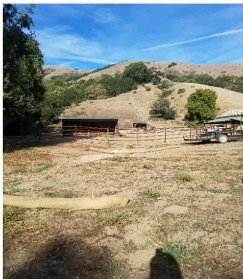
**Figure 4.** Sediment control for areas with concentrated flow
