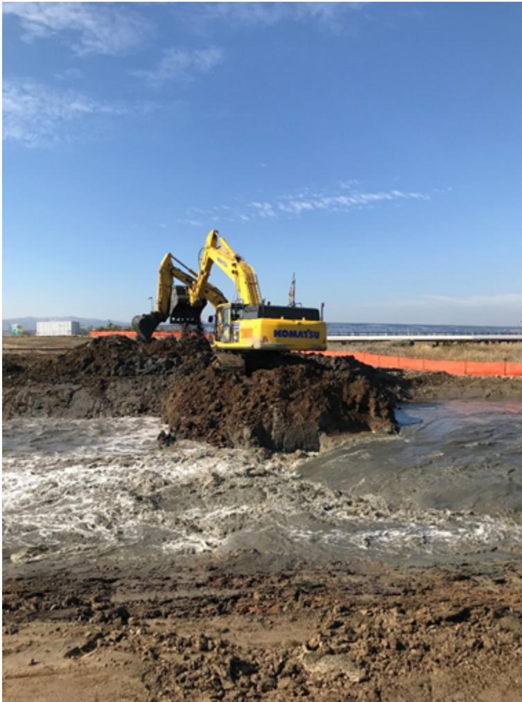
Photo 1. Suisun Bay enters the Project site as two excavators breach the levee.
