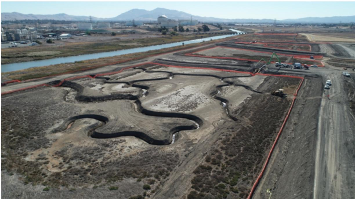
Photo 2. Newly excavated tidal channel network waiting to be connected to Walnut Creek. About six miles of orange fencing was installed and inspected and maintained daily to protect and exclude salt marsh harvest mouse from the Project construction areas.
