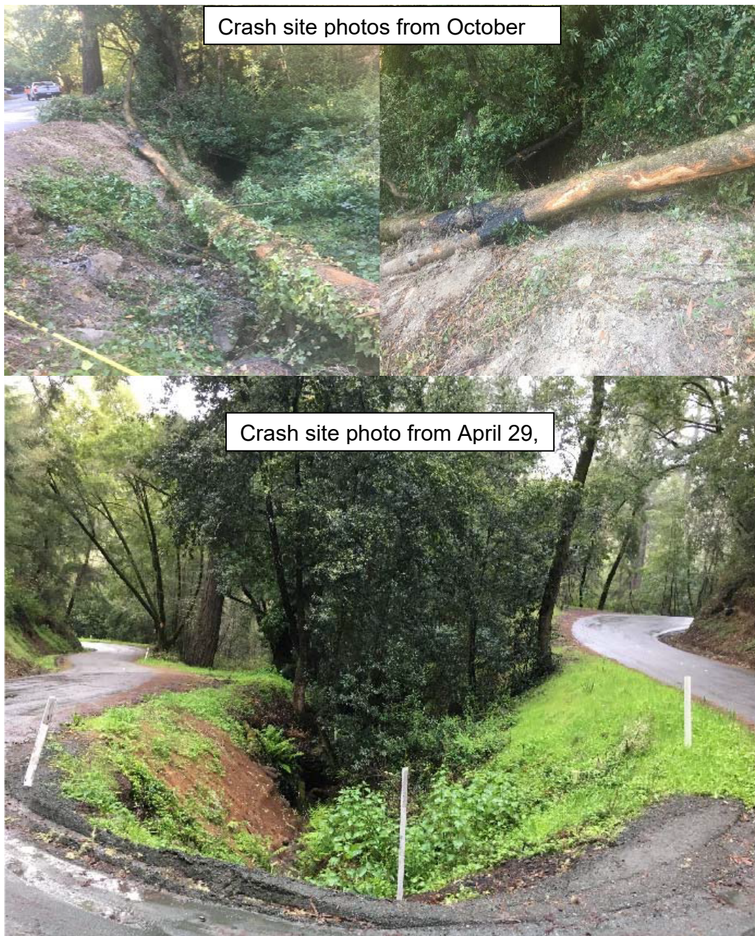
Figure 2. Photos of the crash site from October 2019 and April 2020. Petroleum contamination was excavated to bedrock and stabilization measures were implemented to prevent downstream impacts to the creek.
