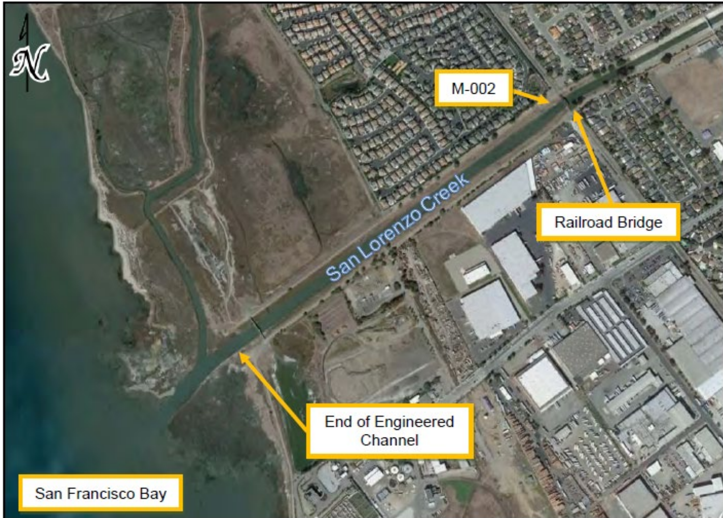
Figure B-2. Aerial View of San Lorenzo Creek Outfall and Surroundings
