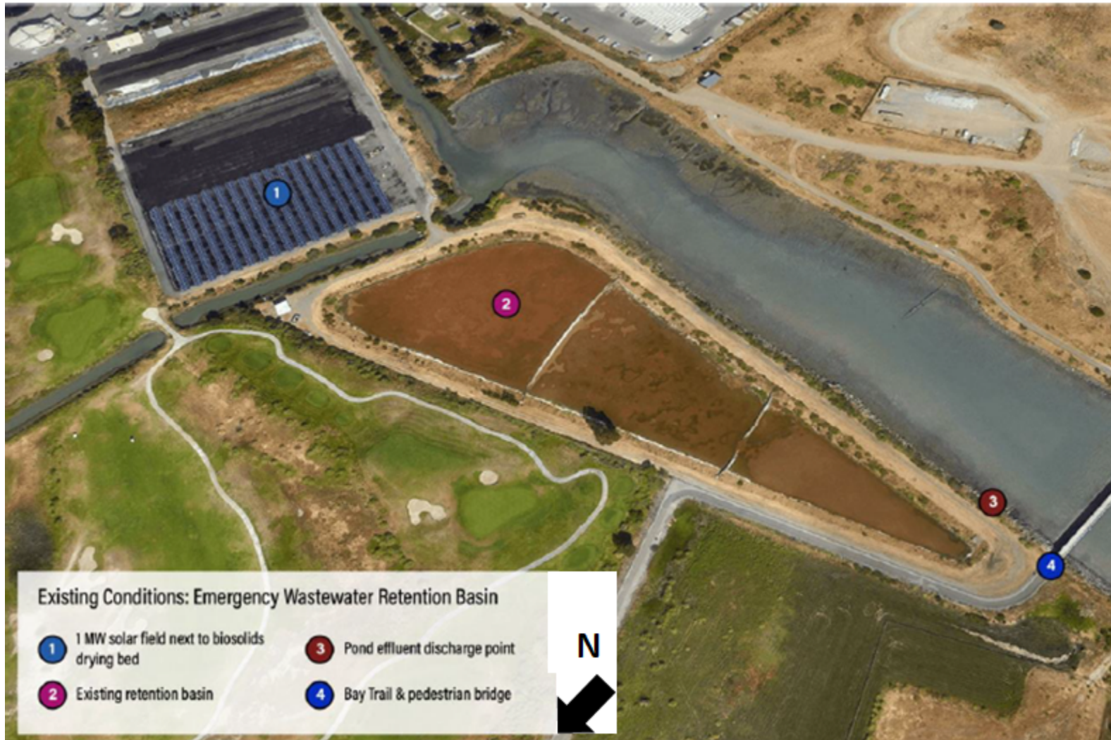
Figure B-2. Aerial View of Existing Storage Basin (Pre-Wetland)
