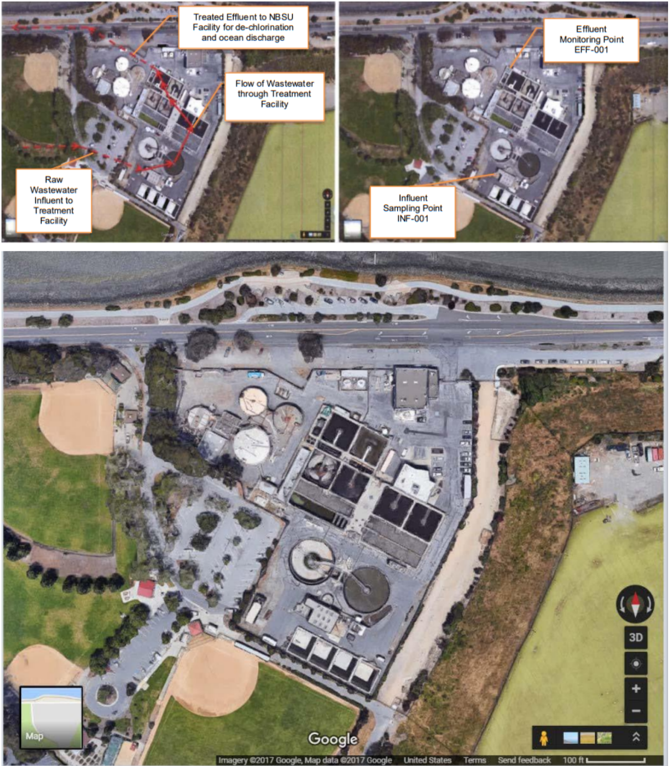
Figure B-2. Facility Aerial View
