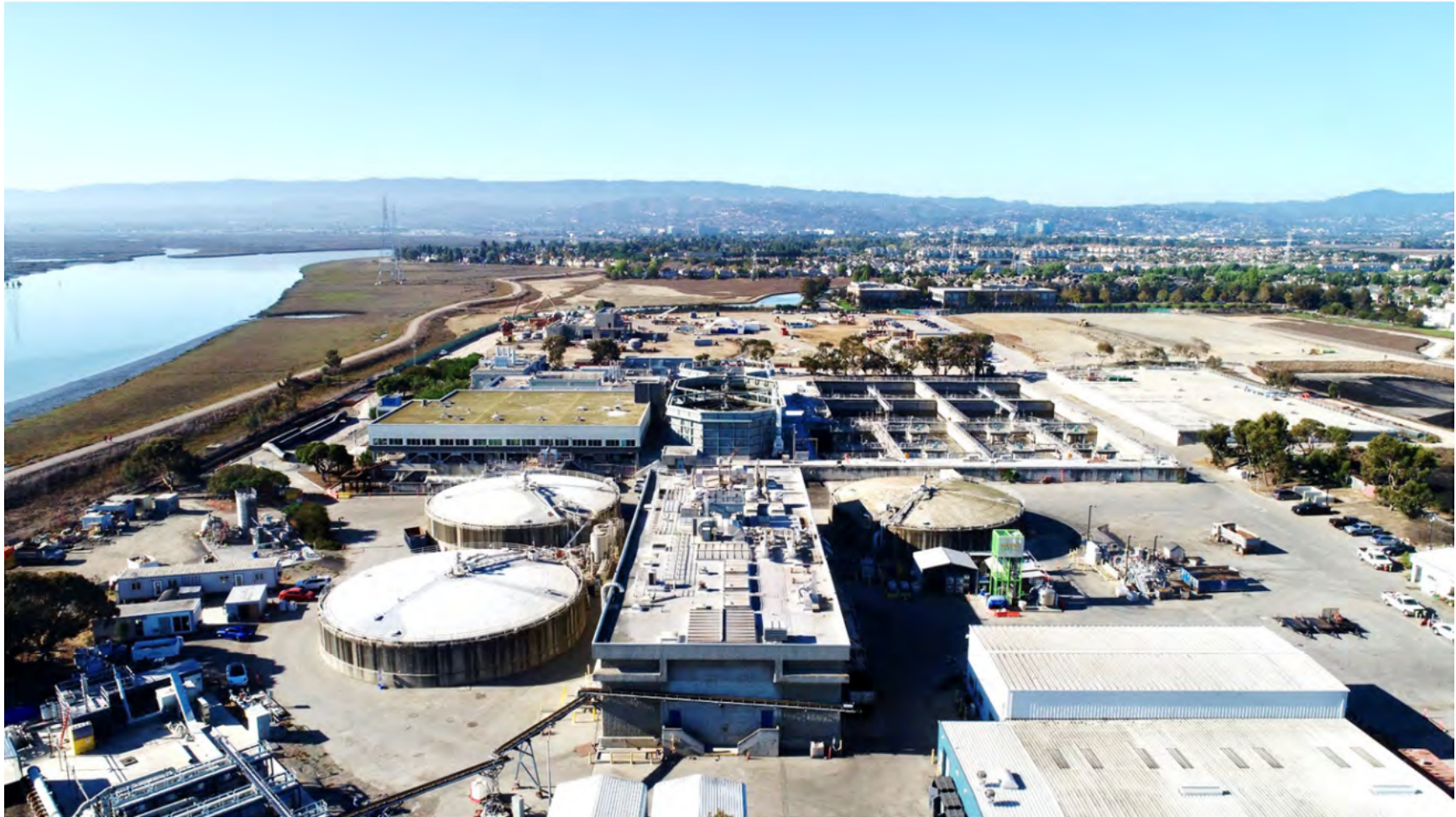
Figure B-2. Facility Aerial View
