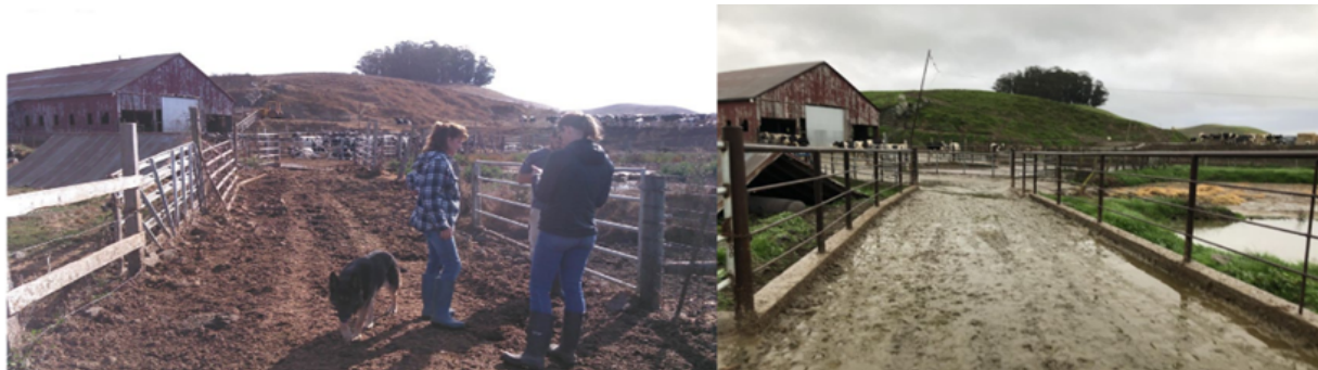
Before (left) and after (right) photos of an improved heavy-use area on a livestock facility. A livestock pathway was upgraded from a dirt walkway to an impermeable concrete path with side walls to prevent pathogen inputs to an adjacent tributary to Laguna Lake in Marin County.
